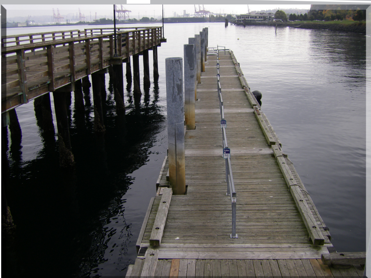
EXISTING FLOATING DOCK
