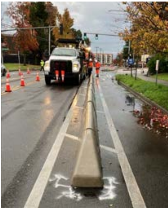
Toronto-style barrier being installed in Seattle
