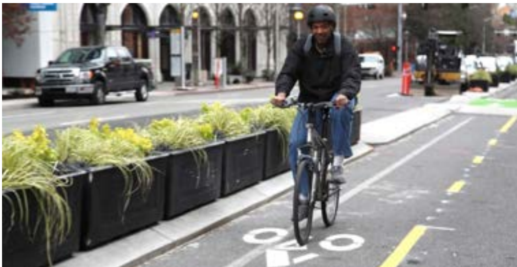
Two-way protected bike lane with planters
