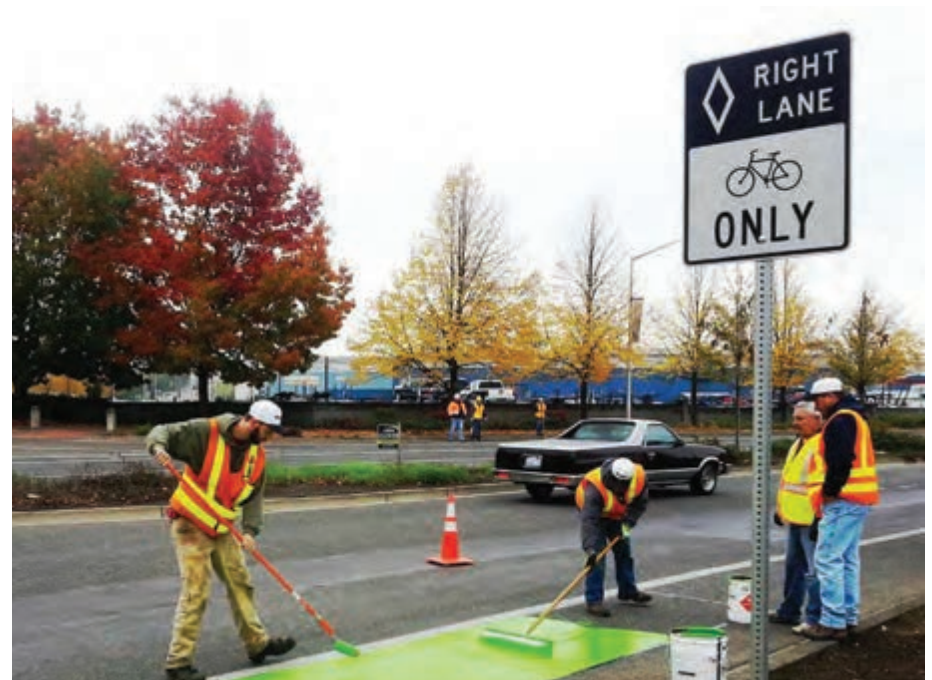
Crews painting a green bicycle lane
