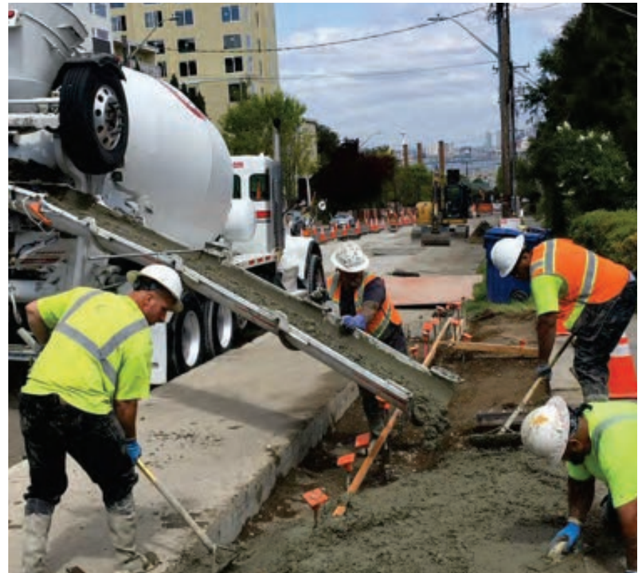
Construction crew at work in West Seattle
