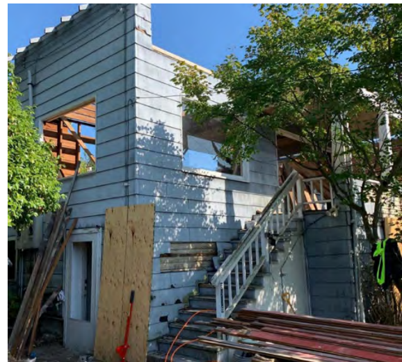
Sledge Seattle deconstructed a house by hand and salvaged lumber for reuse in new construction as part of an SPU grant project. (Source: Sledge Seattle, 2019)
