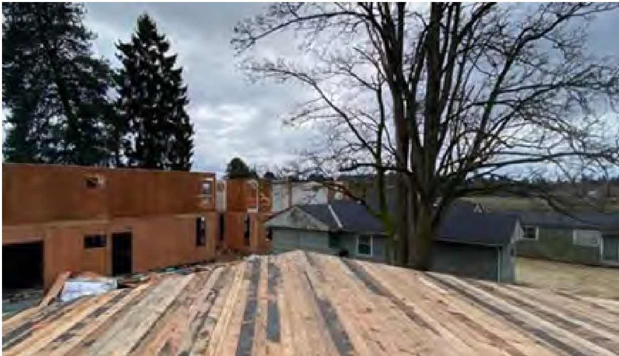
Construction site for three new homes using reclaimed lumber in West Seattle (Source: Seattle Sledge, 2019)
