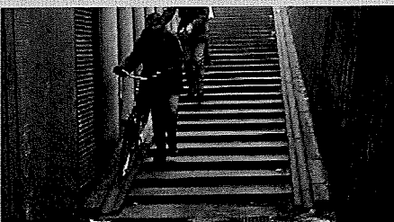
Wheel troughs (bicycle runnels) installed on rail station stairways in Malmo, Sweden
