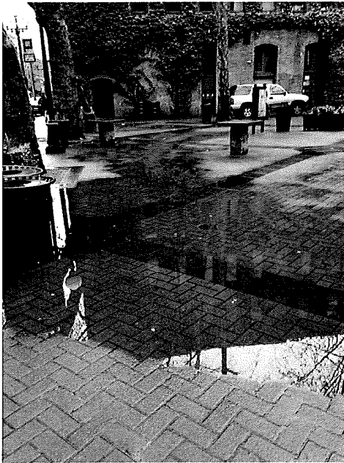
Poor Drainage in the Southwest portion of the park near the information kiosk especially.
