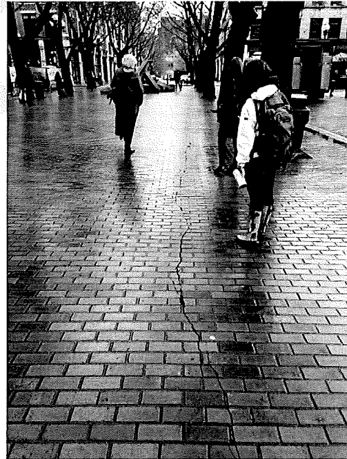
Poor Drainage in the Southwest portion of the park near the information kiosk especially.
