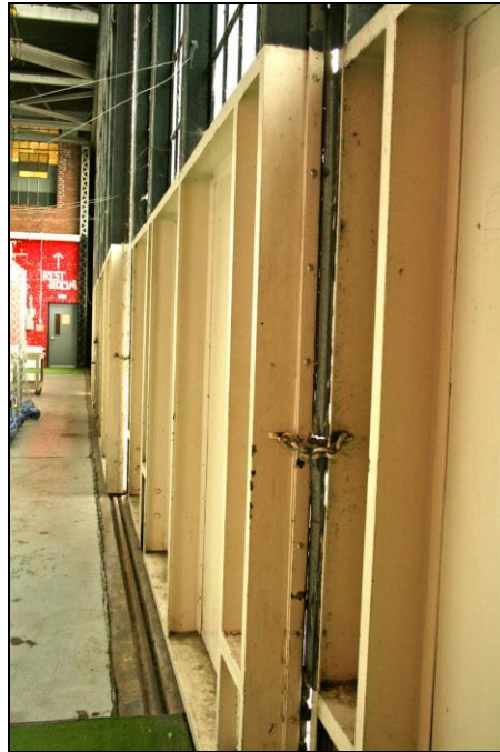
Photo by Megan Espinoza, 2010. North Hangar Interior: Hangar Door Wheel Mechanism (Northern Two-Story Section)
