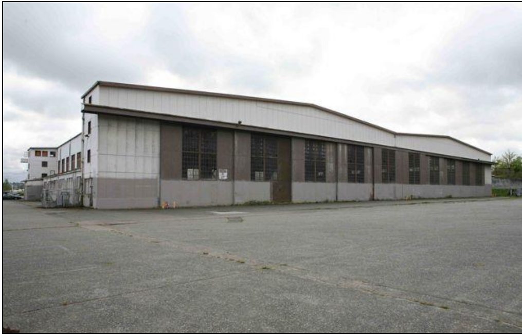
West Facade (Current construction condition)
