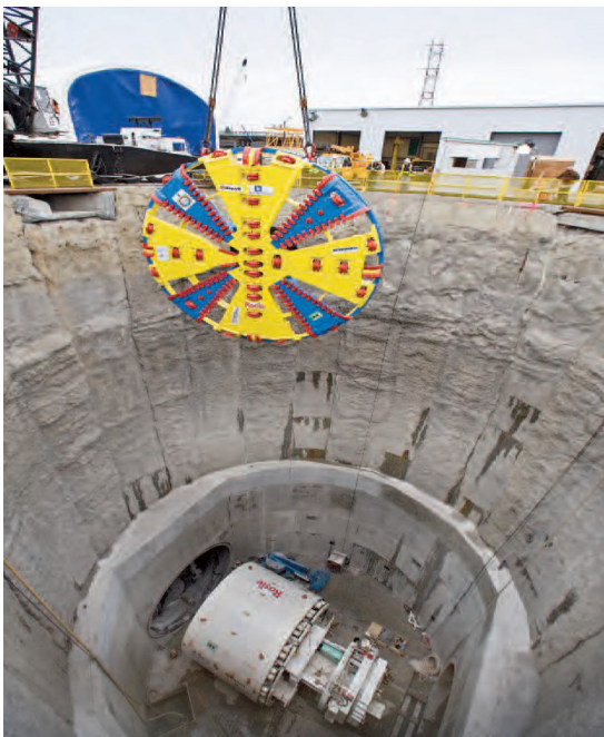
Figure 5-5. Tunnel Boring Machine
