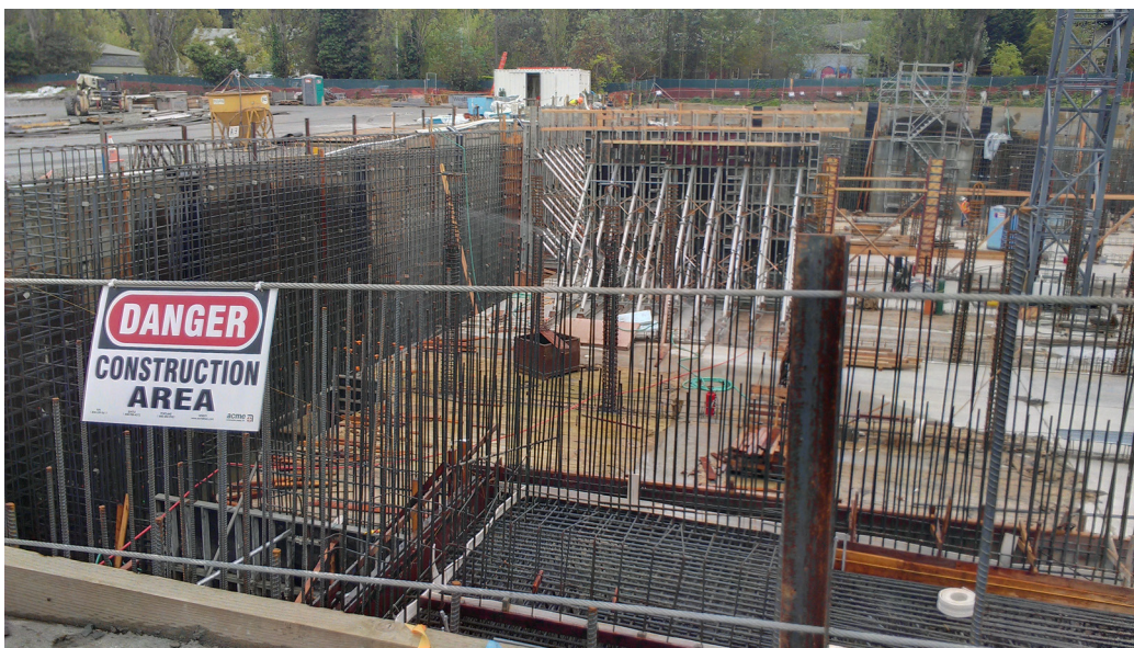
Figure 5-4. Storage Tank Construction
