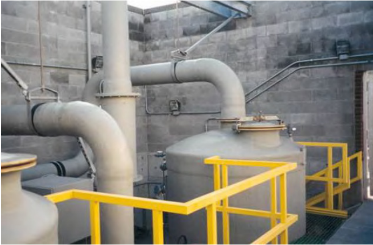
Figure 6-1. Typical odor control equipment for a CSO storage facility
