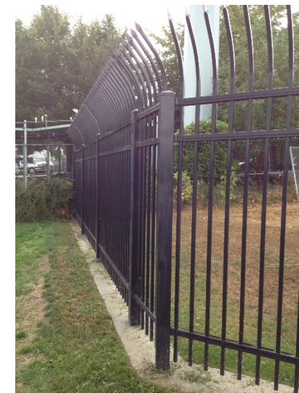
Painted Steel Fence
