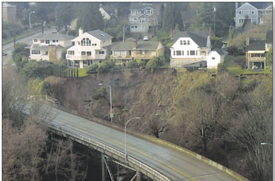
These houses overlook the Magnolia Bridge area of Seattle. The white house on the right side hangs precariously over the headscarp of a large landslide (photo by Hugh Shipman, Washington Department of Ecology).
