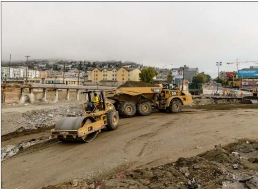
Trucks spread fill dirt before crews pave the roadway.
