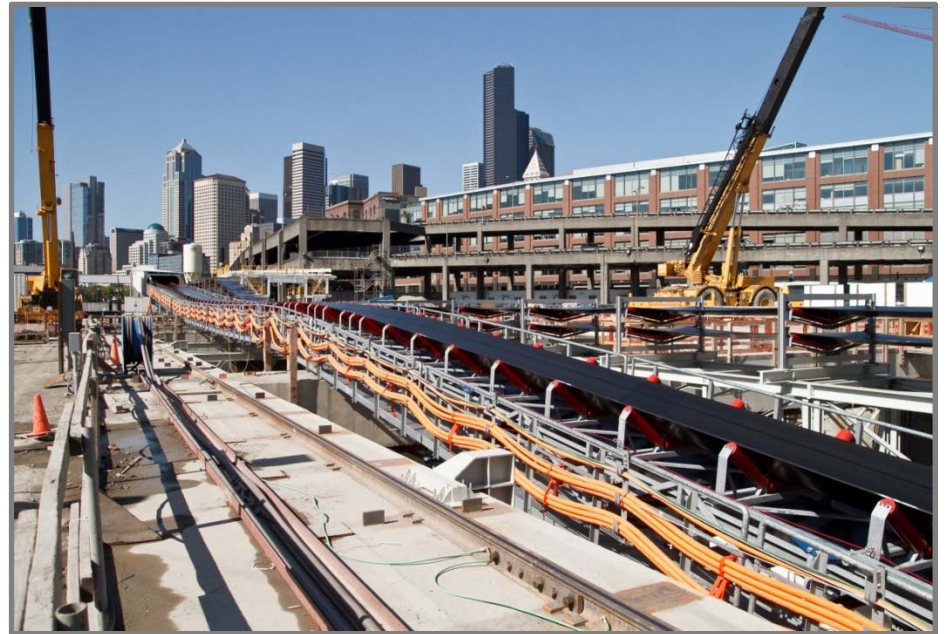
The SR 99 tunnel conveyor belt stretches from the launch pit to Terminal 46.
