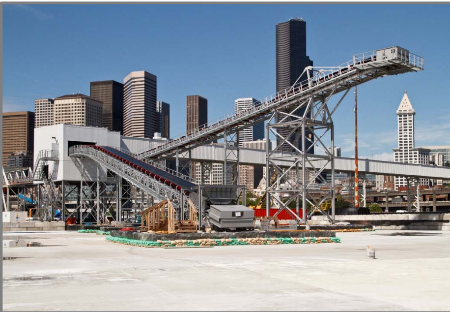
The SR 99 tunnel conveyor belt stretches from the launch pit to Terminal 46.
