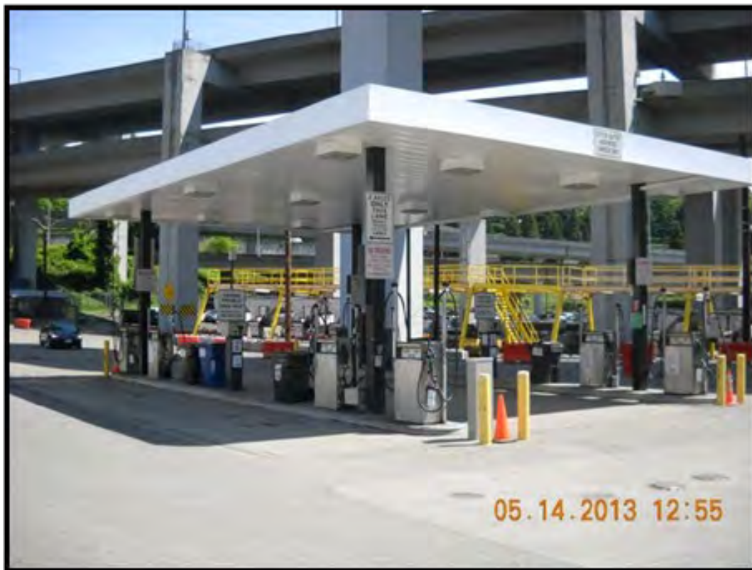
Figure 48. Roof at Fueling Island to Prevent Stormwater Run-On.
