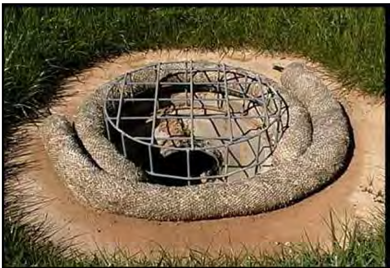
Figure 17. Straw Wattles or Compost Sock for Inlet Protection.
