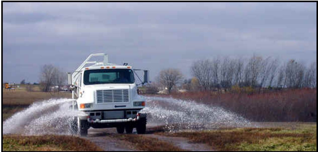
Figure 11. Using a Water Truck for Dust Control.
