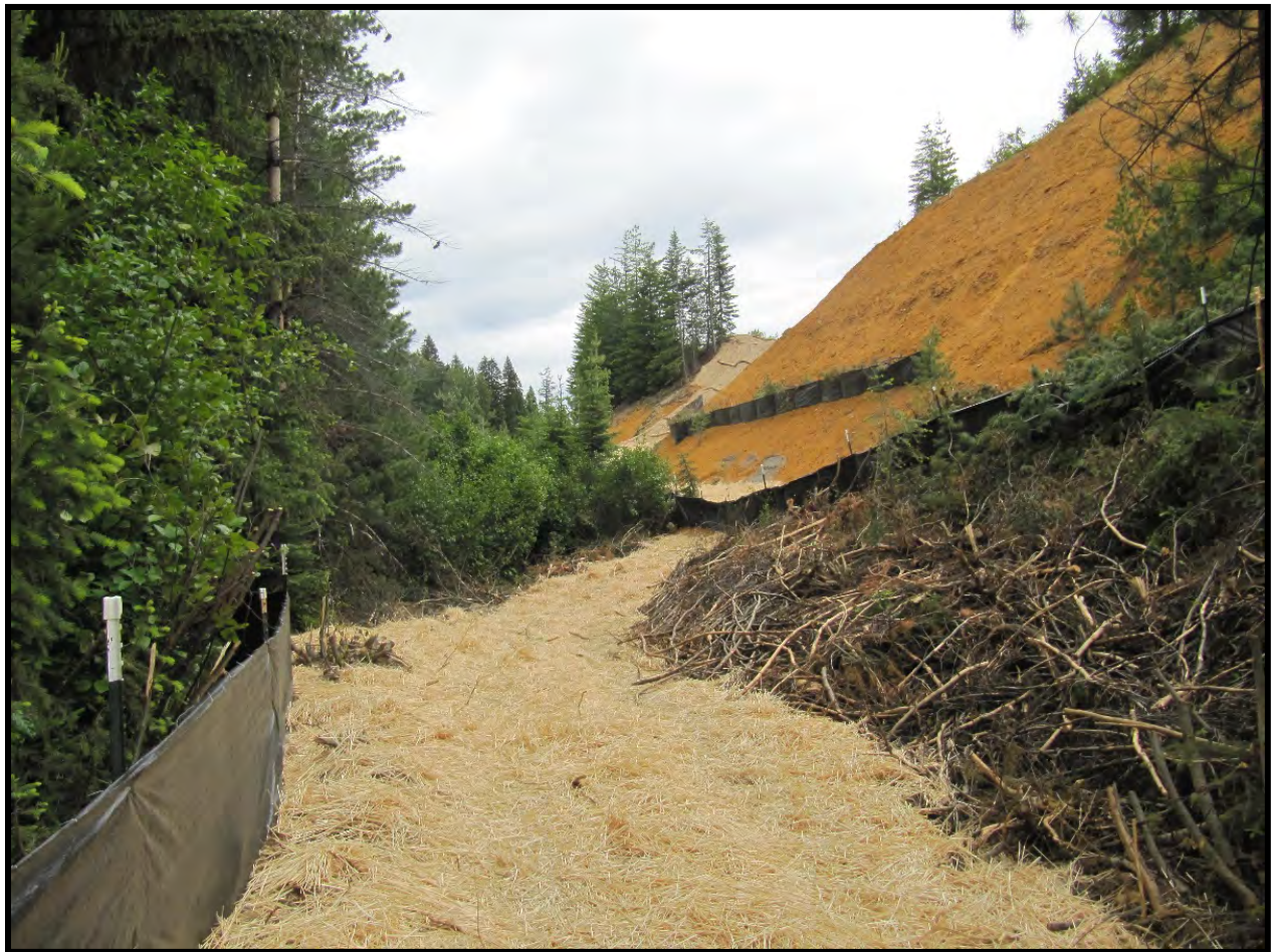
Figure 13. Filter Fence Installed on a Slope.
