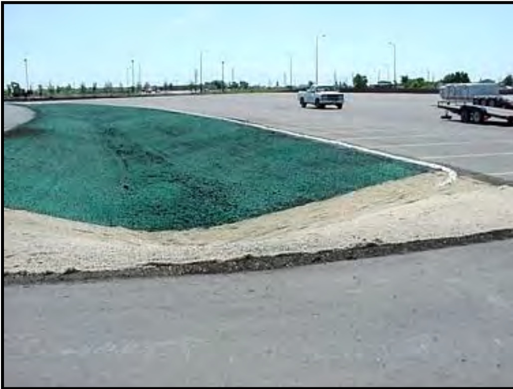
Figure 1. Hydroseeding Method.
