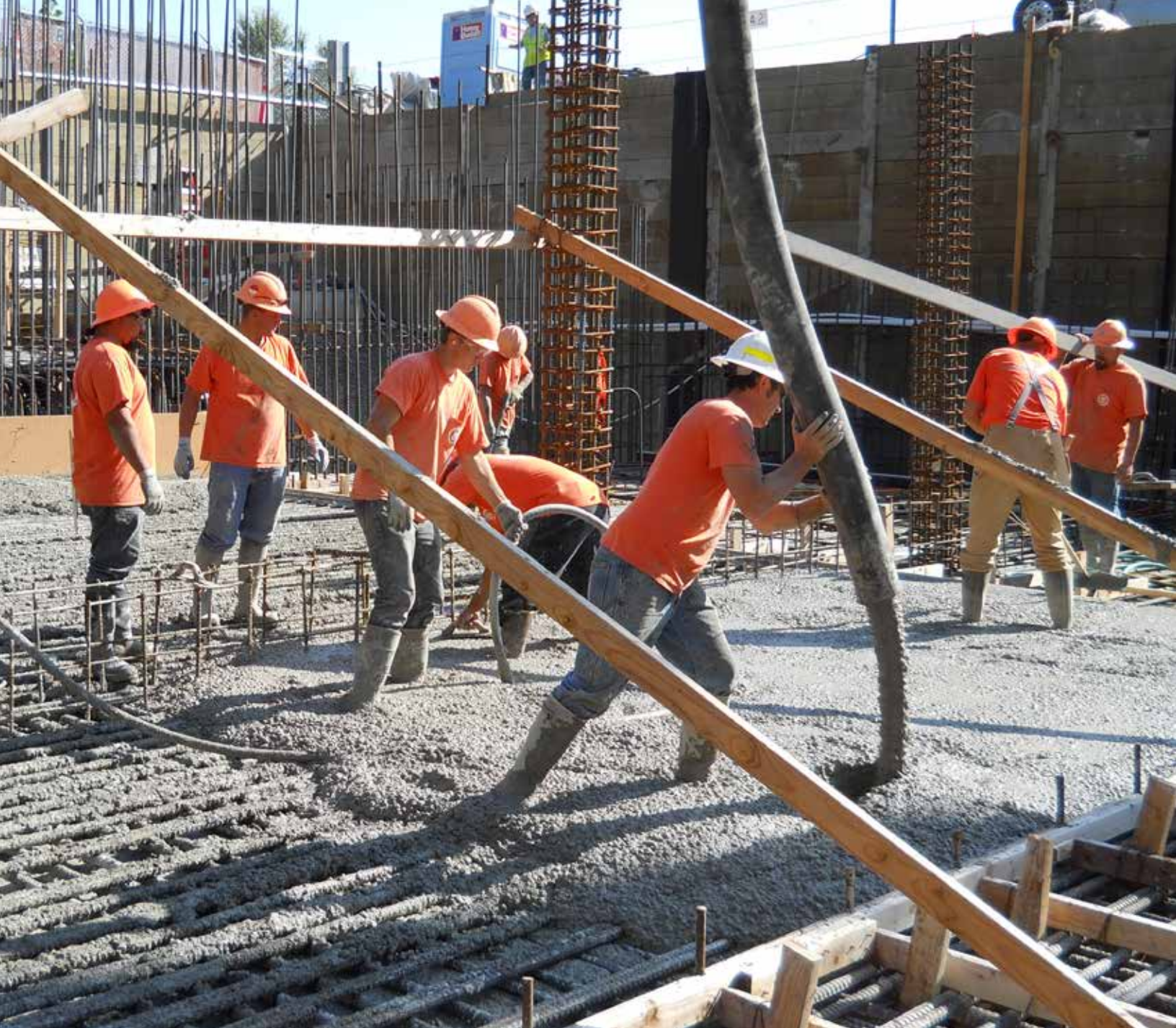
Pouring the foundation for a 2-million-gallon storage tank to keep pollution from reaching Lake Washington.
