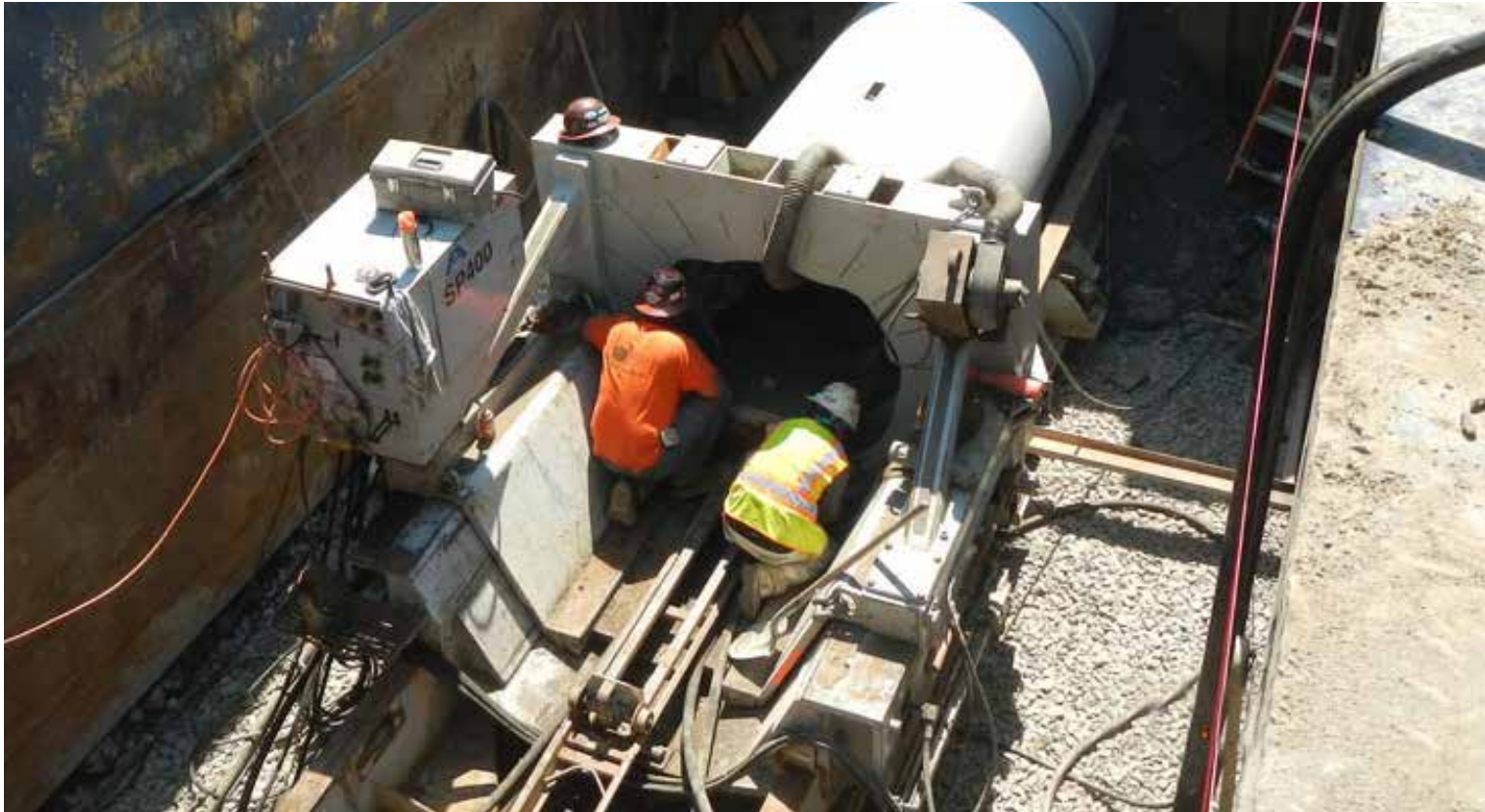
Installing a new section of pipe for the Madison Valley Stormwater Project.
