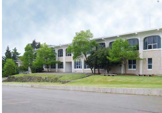
Figure 14: View of Leisy USARC Building 220 South Elevation
