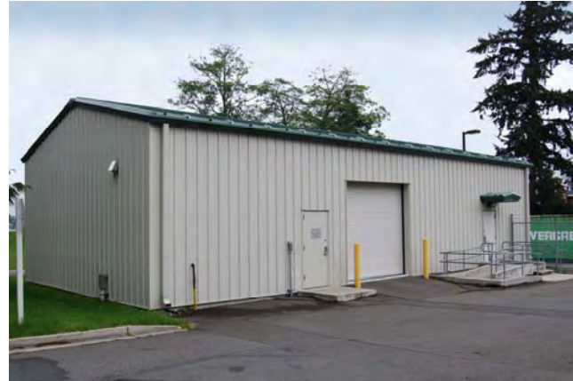
Figure 5: Exterior View of Building 214
