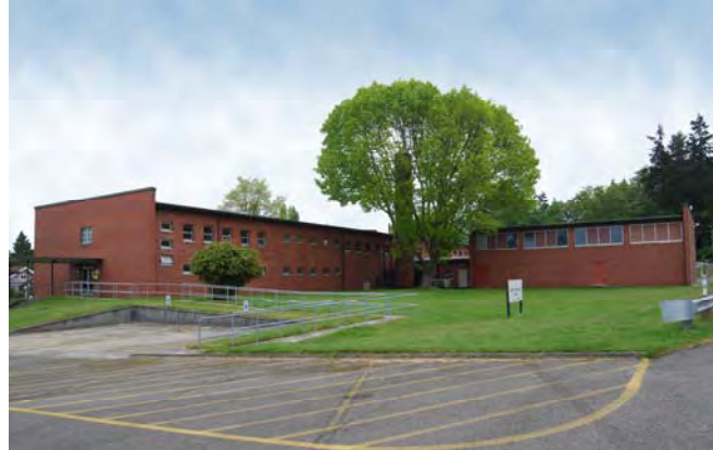
Figure 9: View of Harvey North Elevation
