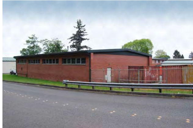
Figure 2: Exterior View of Building 211
