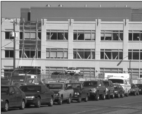
Adaptive Reuse - light industrial-style large windows, parapet, building facade broken up by vertical elements to reduce the scale
