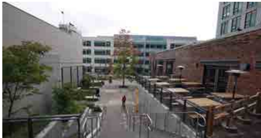
Capitol Hill Transit Oriented Development
