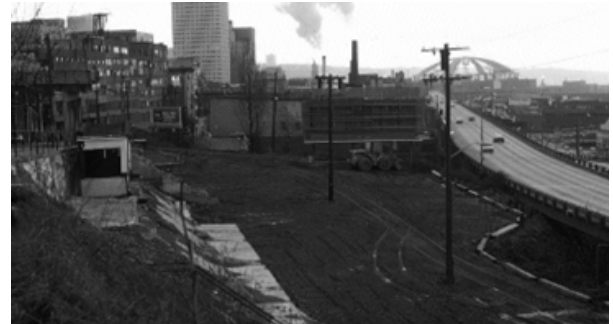
Site cleared and graded for surface parking, 1974
