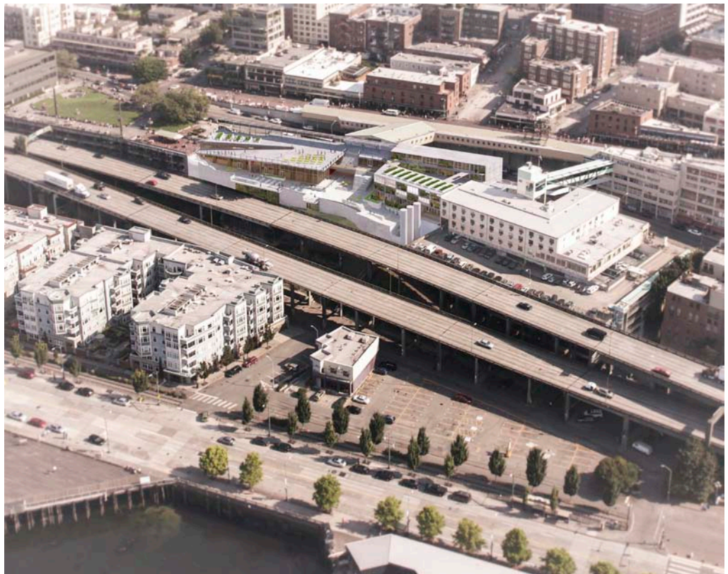
Site Phasing #2: Construction of PC1N complete, Fall 2015
