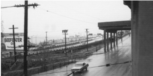
Site cleared and graded for surface parking, 1974
