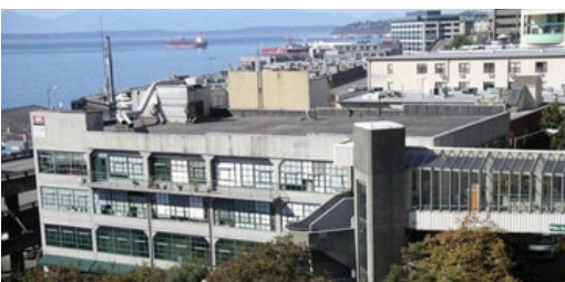
Concrete frame with glass infill
