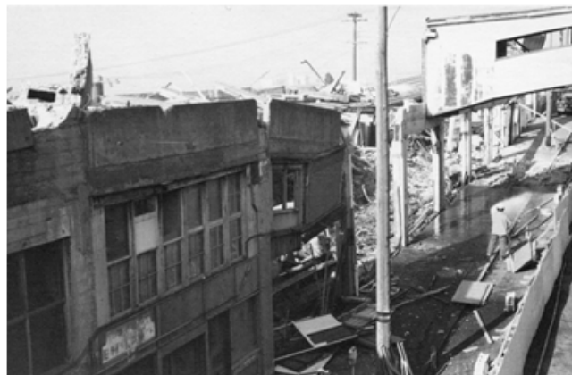
Municipal Building being demolished after the fire, 1974
