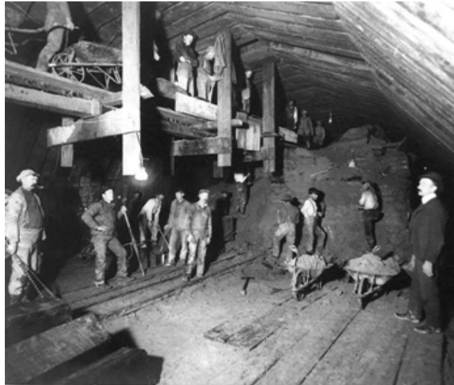
Crews excavating and placing timber shoring, 1903
