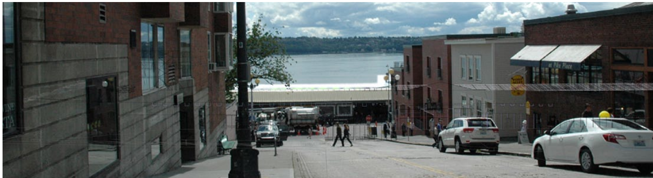
View of project from Stewart St.
