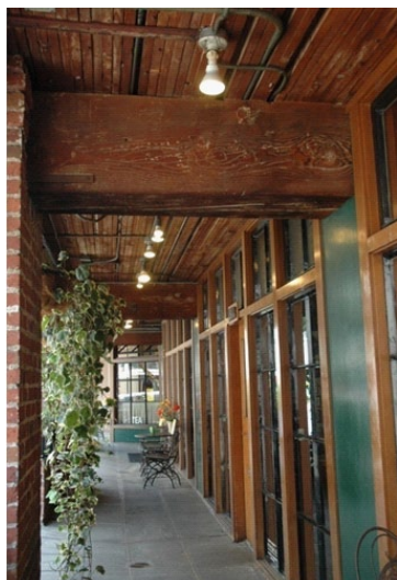
Heavy timber framing
