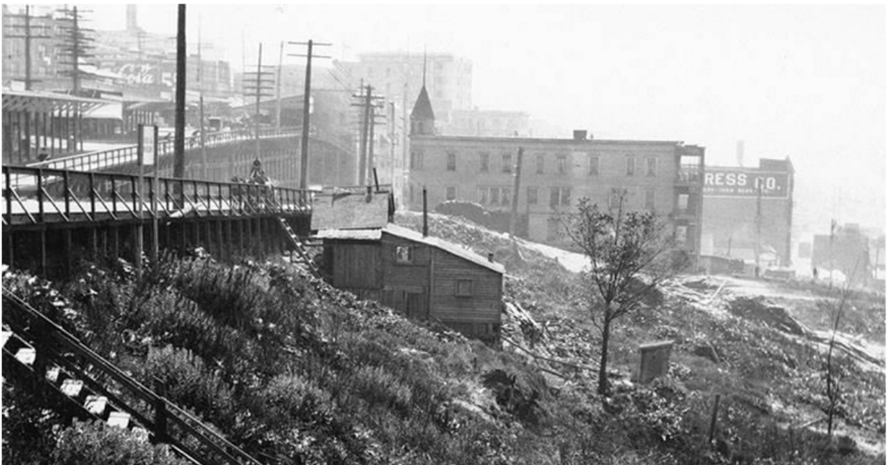
View across site to the south, 1909
