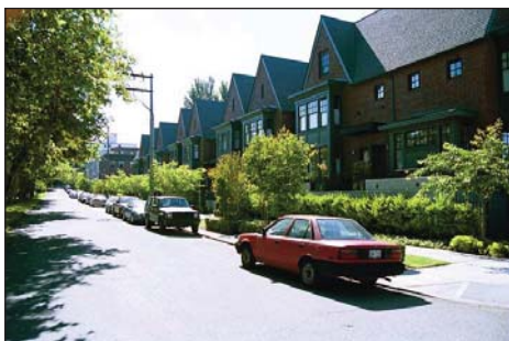
Victoria Townhouses (Comstock Street, Queen Anne). The use of traditional pitched roofs, gables, and bays achieves a scale and character consistent with the neighborhood.
