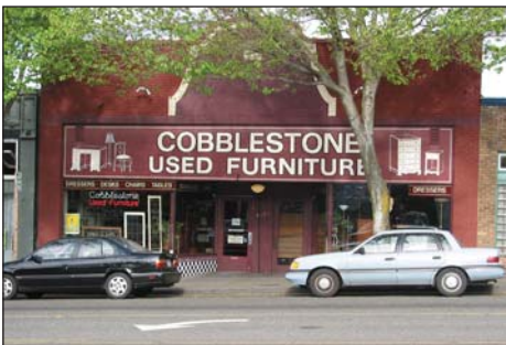
Cobblestone Used Furniture (Greenwood Avenue North between North 84 th and North 85 th Streets). Again, a modest scale and traditional storefront features make this a good example. The decorative tile use, inset entry, and display windows add interest. Although the sign is large, its detailing and execution make it appropriate in its context.
