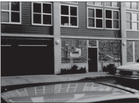
The parking in this structure has been integrated into the overall building design in a cohesive manner and is further concealed through decorative metal grille work
