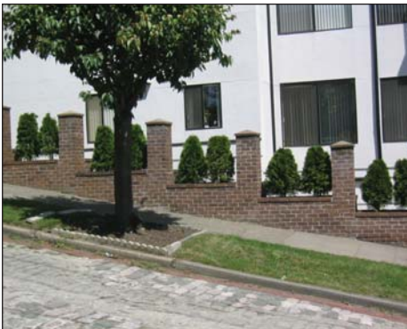
Retaining walls constructed with durable materials and landscaping soften the building edges along these two sloping streetscapes.
