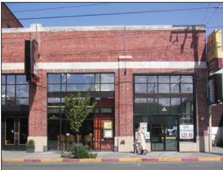
A regular cadence of storefront windows and pilasters along the street-level facade enhances the pedestrian experience.
