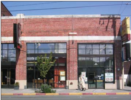
A regular cadence of storefront windows and pilasters along the street-level facade enhances the pedestrian experience.
