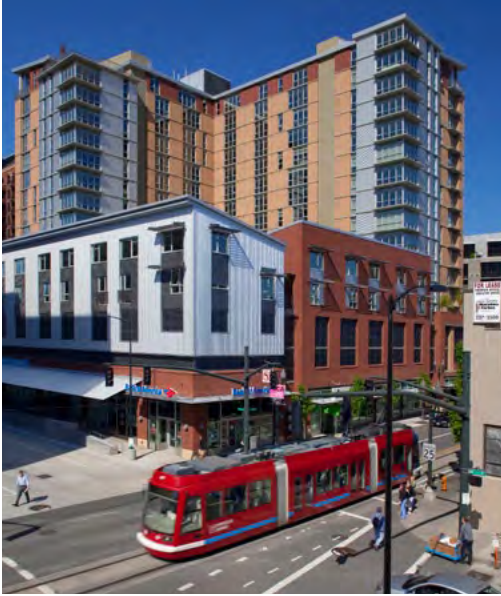
Differentiated massing and housing types This building incorporates highrise flats, courtyard-level townhouses, concealed parking, and street-level retail, all within a single block. Massing and facade design differentiate the housing types, reduce the bulk of building, offer a consistently activated street-edge, and create a balanced formal composition of the block. (Photo: Gregg Galbraith; Design: GGLO)
