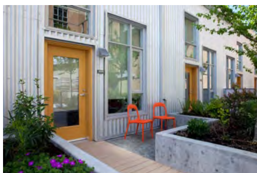
Ground-level entries The setback entrance to an individual residential unit clearly marks the entry, and provides usable private outdoor space that successfully transitions a resident or visitor from the public to the private realm. (Photo: Gregg Galbraith; Design: GGLO)
