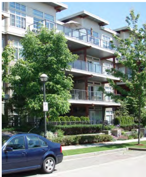
High-density residential frontage These family-sized units, organized as stacked flats, have relatively large yards and decks, all overlooking a neighborhood street. (Photo: Don Vehige)
