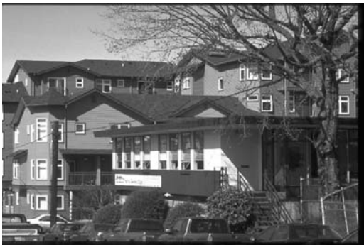
The roofline of this large development adds to the structure's residential identity and reduces its apparent bulk.
