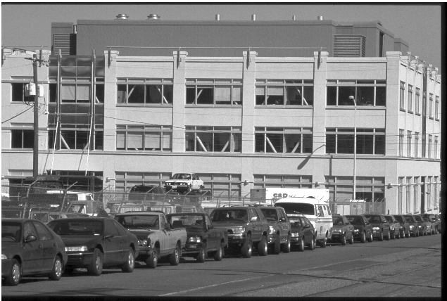
Adaptive Reuse - light industrial-style large windows, parapet, building facade broken up by vertical elements to reduce the scale
