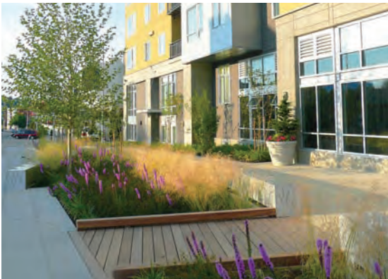
Rain gardens infiltrate stormwater runoff at Taylor 28, a new mixed-use multi-family housing project at the corner of Denny Way and Taylor Ave in SLU. Photo: Dan Bertolet
