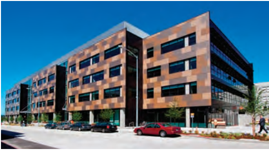
Completed in 2010, this mixed-use office building located on Boren Ave N between Mercer and Republican Streets provides 158,000 square feet of office for Amazon.com, along with 14,000 square feet of street level retail.
