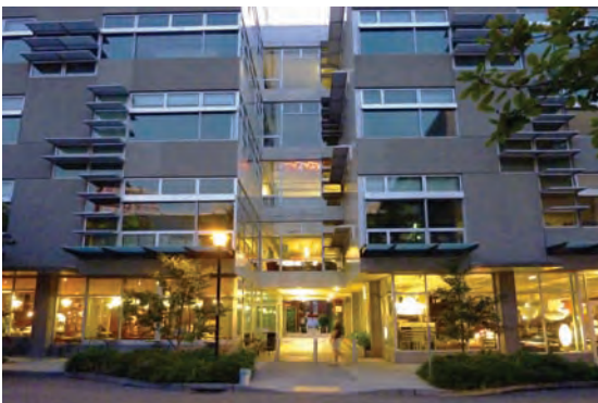
Alley 24, a full-block mid-rise development located adjacent to REI in SLU, is one of the City's best examples of true mixed-use development, providing office, retail, and rental housing, with 20 percent of units affordable to households earning less than 60 percent of area median income. Photo: Dan Bertolotto
