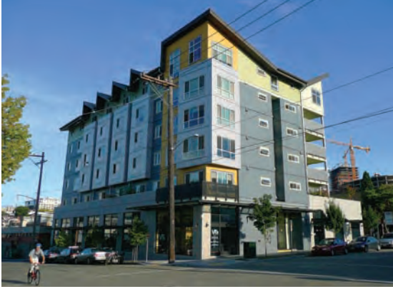
The Denny Park Apartments in SLU, completed in 2005, provide 50 units affordable to households earning 30, 50 and 60 percent of area median income. Photo: Dan Bertolet
