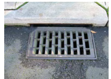
Typical storm drain
