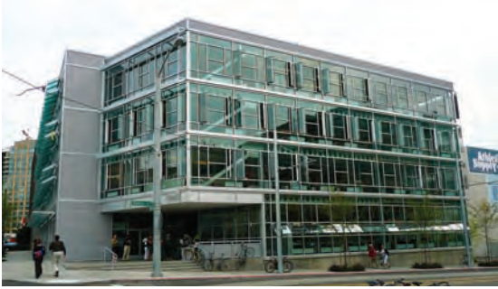
The Terry Thomas office building in SLU, completed in 2008, incorporates passive heating/cooling strategies, which eliminate the need for air conditioning, and will lead to an estimated 30 percent reduction in energy use. Photo: Dan Bertolet
