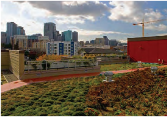
Green roof on the Bart Harvey, an apartment developed by the Low Income Housing Institute in 2010 that provides 49 units of affordable housing for low-income seniors. Photo: Michael Seidl
