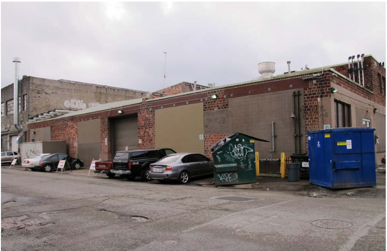
East elevation (facing Occidental Street)
