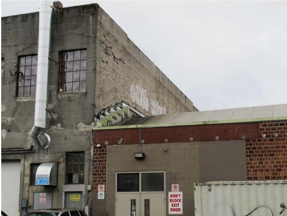
Partial view of north party wall
