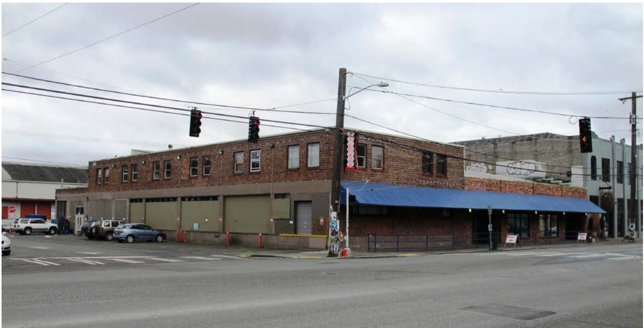
View from the northwest
