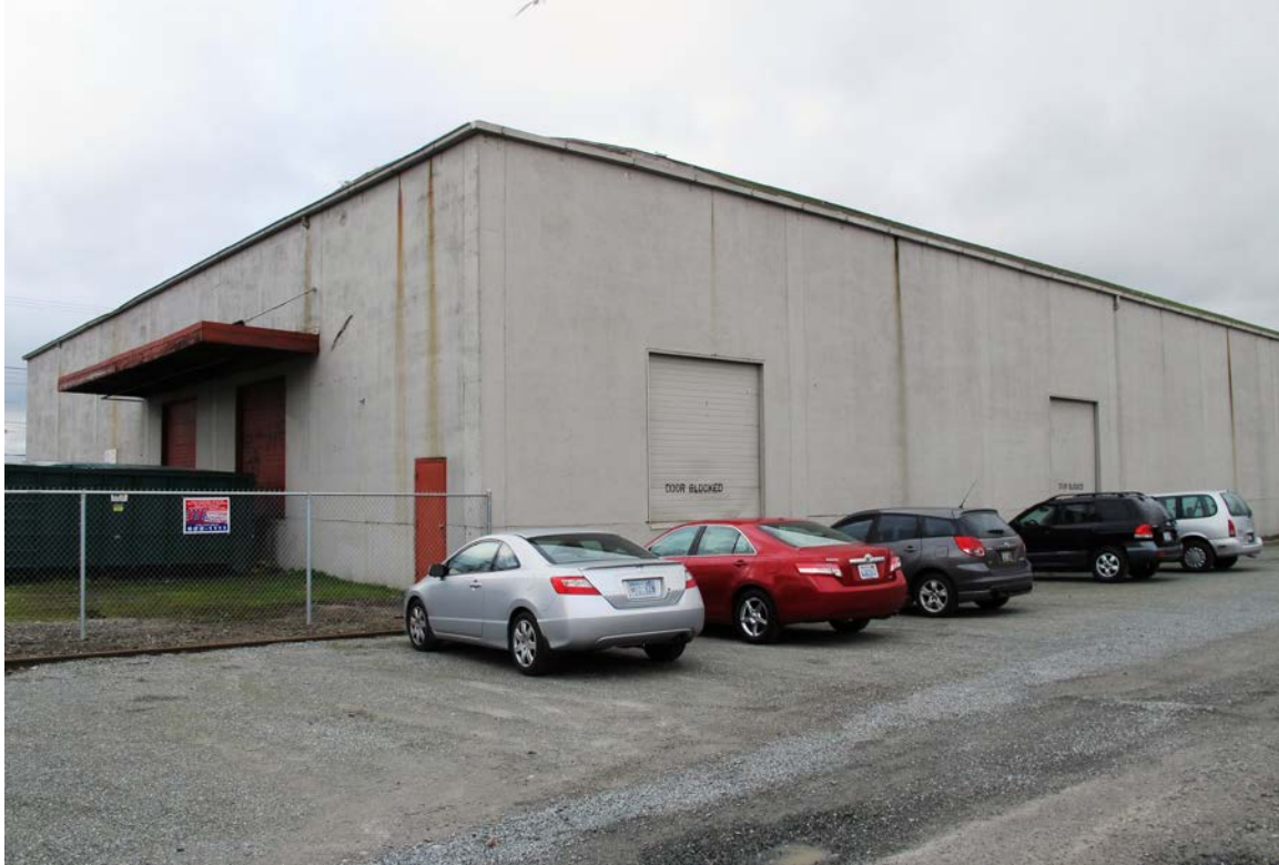
View of south (left) and east (right) elevations
