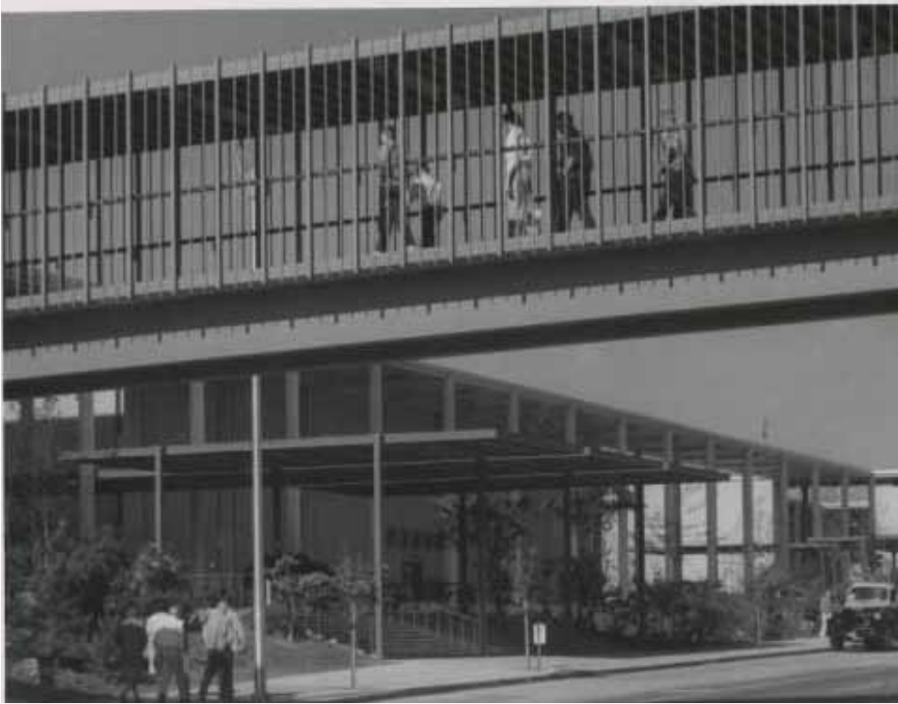
Historic image of skybridge crossing over Mercer Street from the Mercer Street Parking Garage to the fair site. Source: Seattle Public Library.
