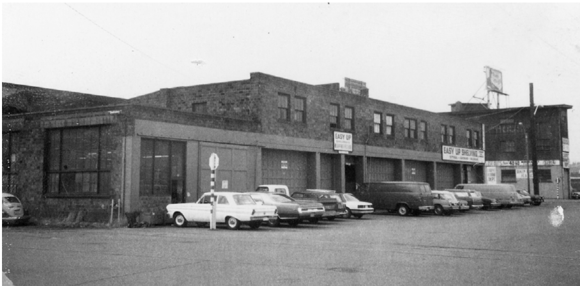
1980 tax assessor photo, north elevation (from northeast). Compare to 2013 photo; note alterations to loading bays.
