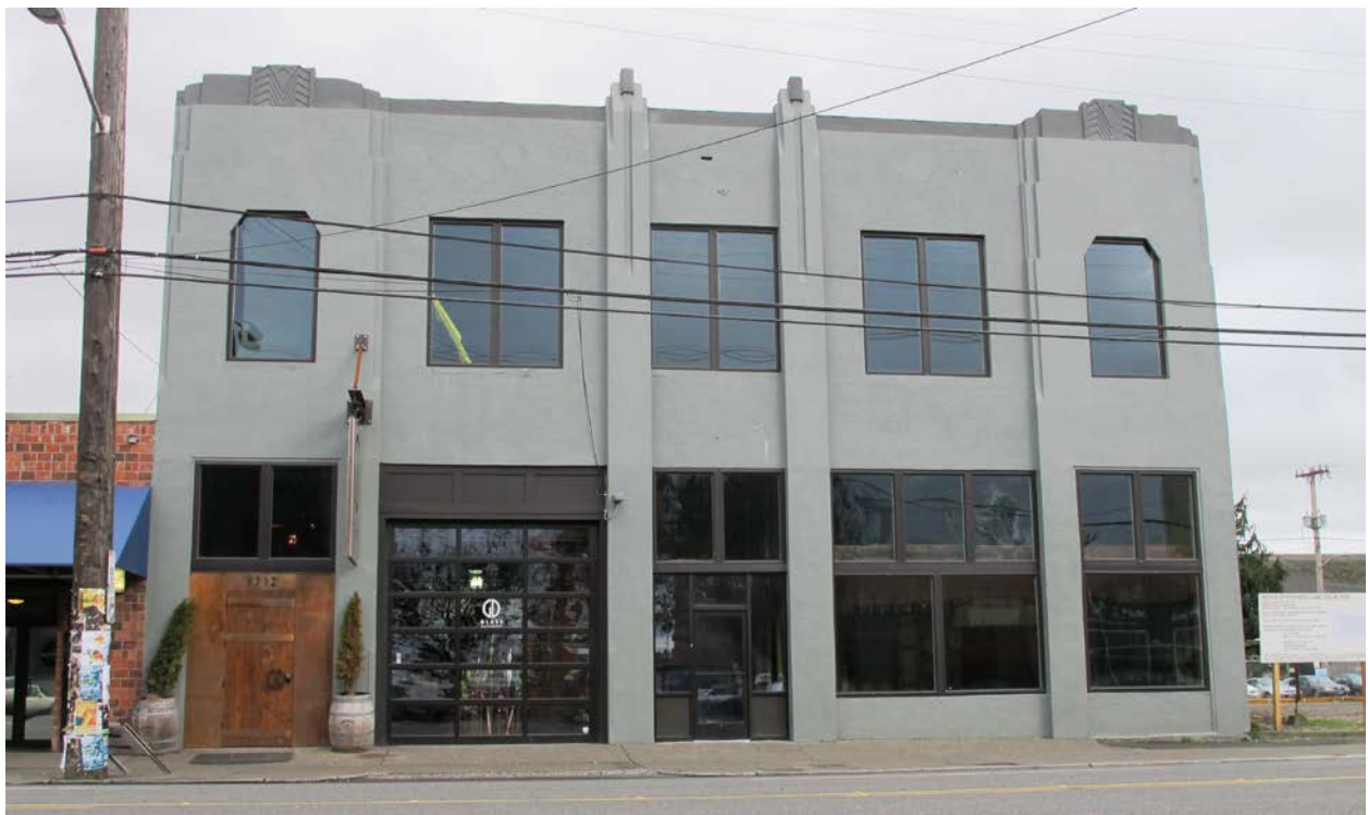
West elevation (facing First Avenue S.)
