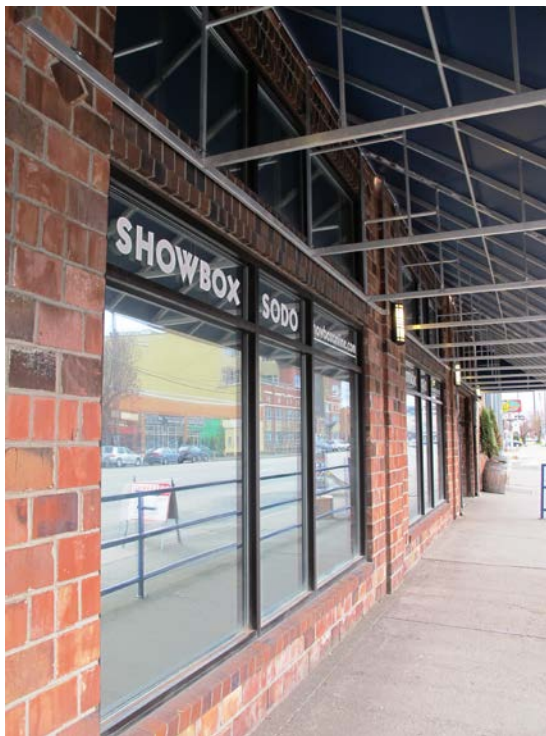
Detail, west elevation (facing First Avenue S.). Diamond-shaped tiles, shaped window headers, windows, and light fixture are non-original and date from a 2003 renovation. Compare to 1937 tax assessor photo.
