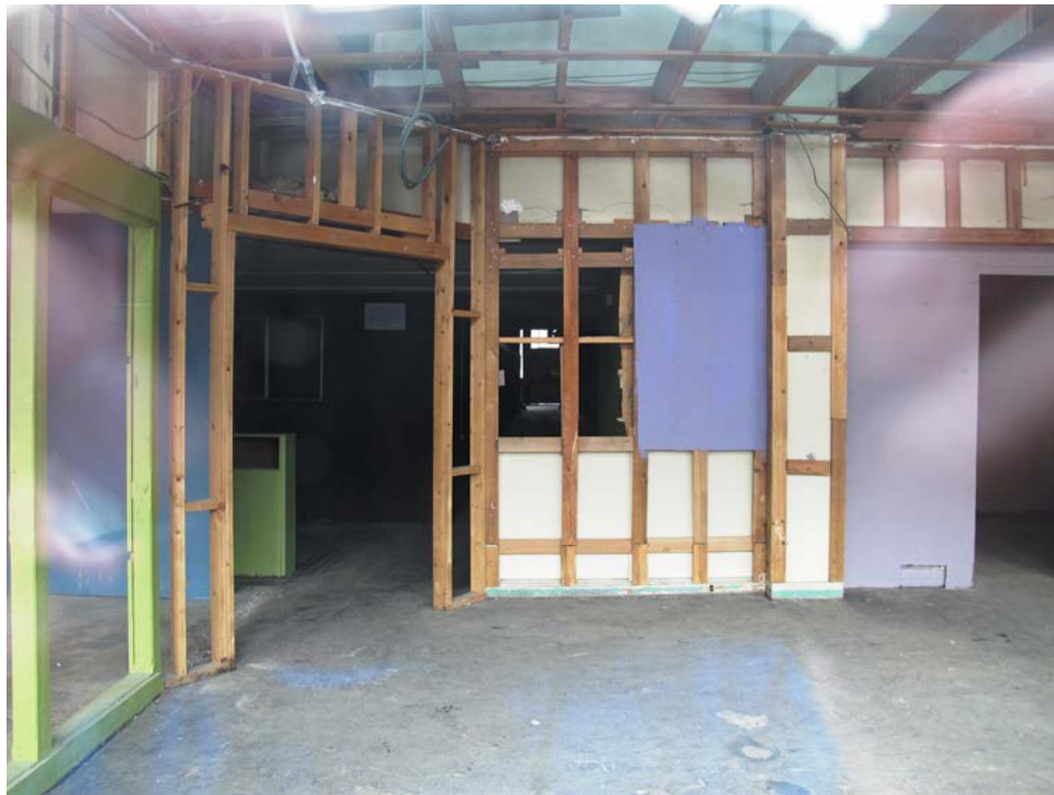
View into storefront at sidewalk level, south side of main elevation.
