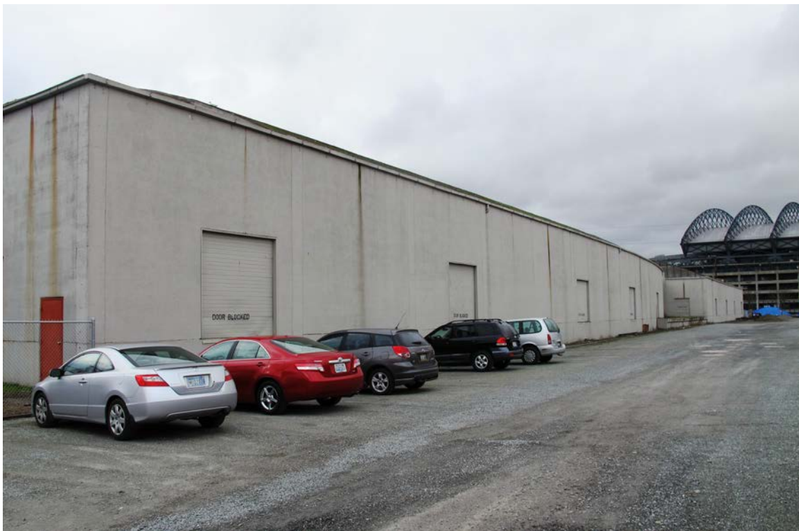
Looking northward at the east elevation
