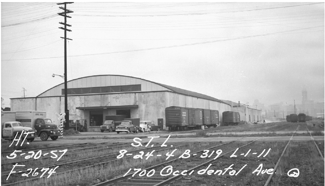
1957 tax assessor photo of original building (foreground) after construction of the addition (visible in the distance), showing south elevation (facing S. Holgate Street) and east elevation (facing railroad tracks).
