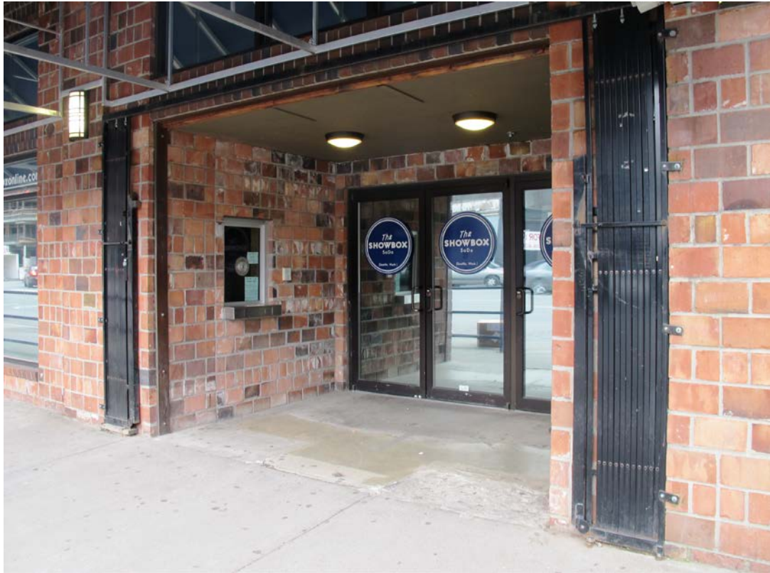
Detail, west elevation (facing First Avenue S.), showing main entrance.
