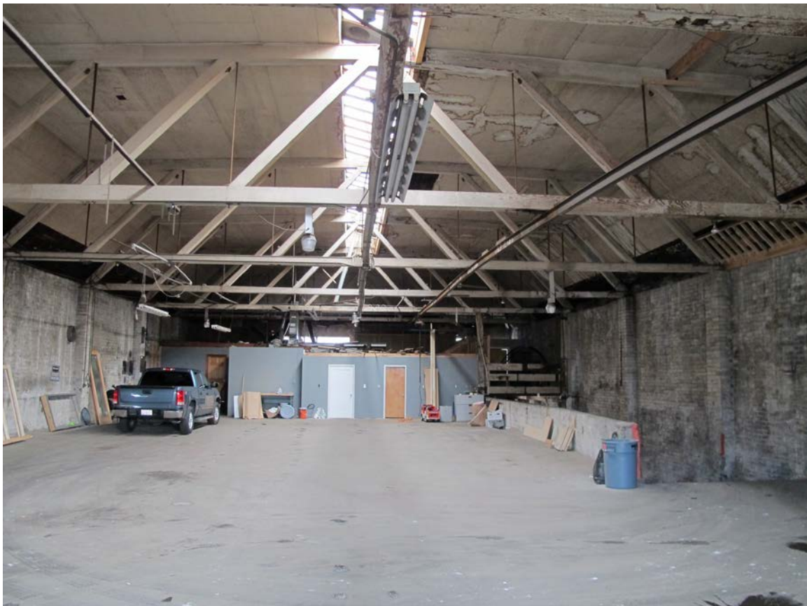
Second floor, southern half of the building (top of ramp).
