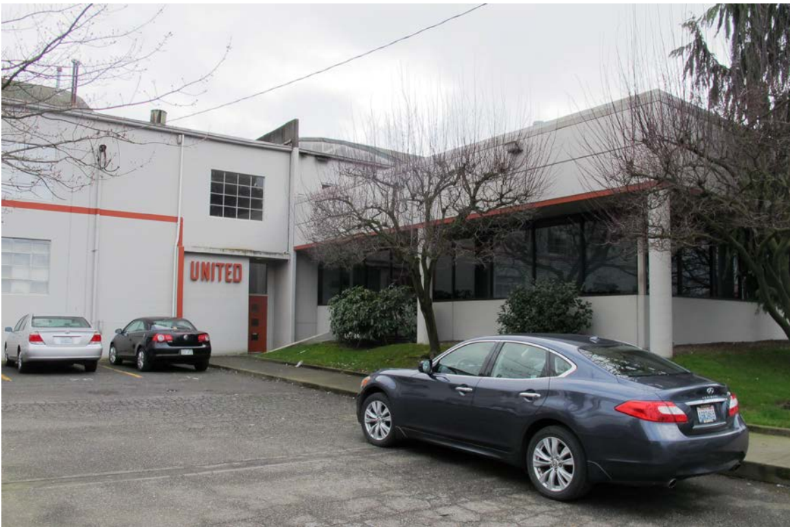
West elevation, midblock, showing office addition at right.
