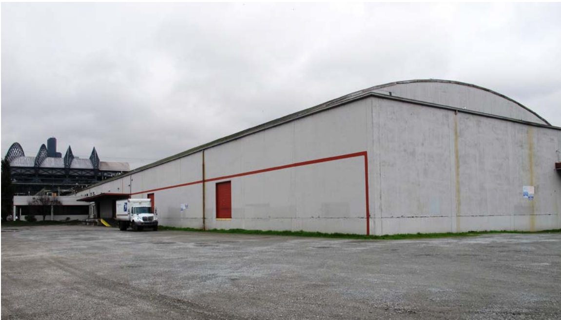
Looking northward, on Occidental Avenue S. at corner of S. Holgate Street, at the west and south elevations. Note office addition at far left.
