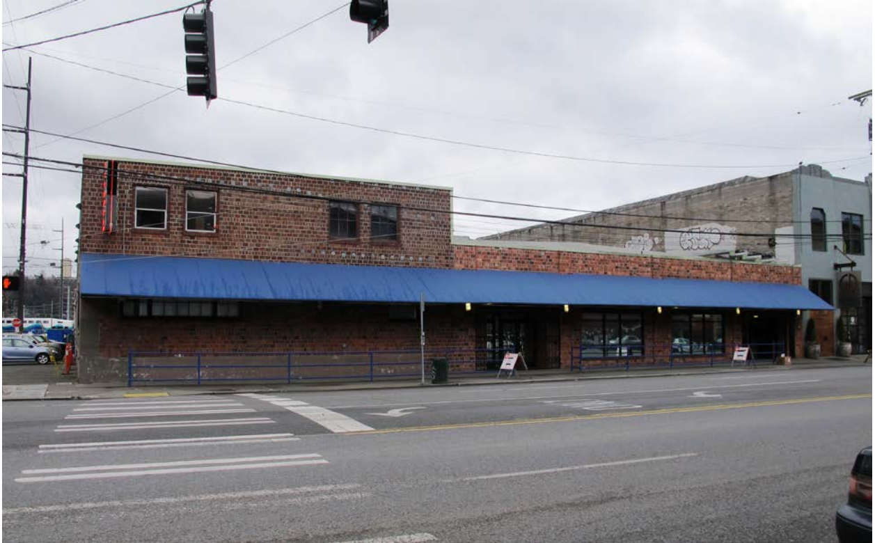
West elevation (facing First Avenue S.); note alterations to the right side of the facade (compare to 1937 photo).
