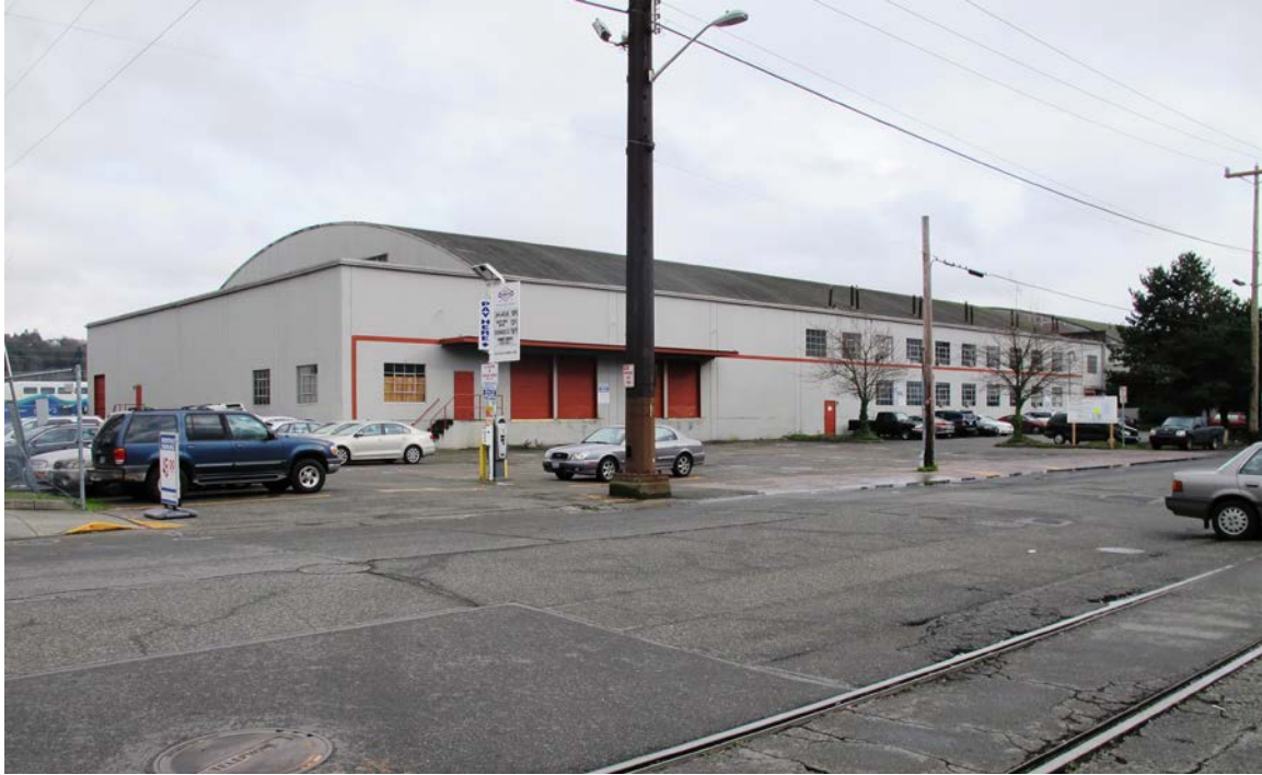
North elevation at left (facing S. Massachusetts Street), west elevation (facing Occidental Avenue S.) at right.
