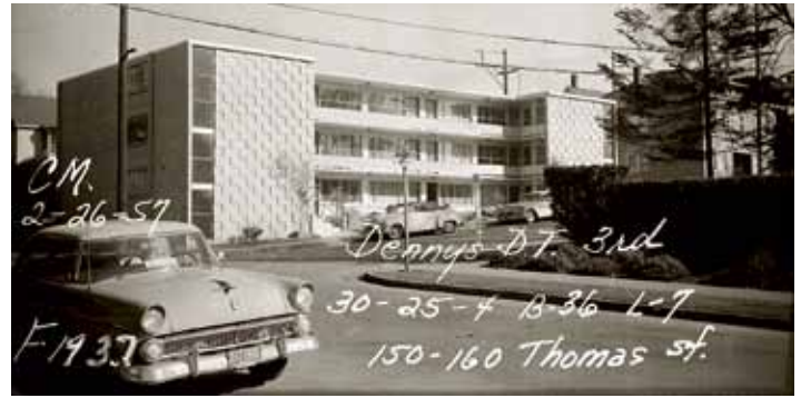
1957 image of the Blue Spruce Building (Blue Spruce Apartments, Administration Building). Source: Puget Sound Regional Branch, Washington State Archives.
