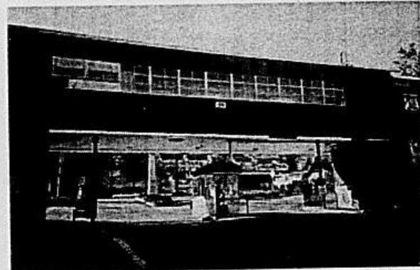
Photo 4.2.53 Building 138 east facade showing guard house in roadway
