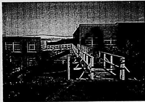
Photo 4.2.13 Bridge addition for roof access Building 5
