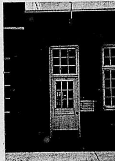
Photo 4.2.25 Building 11 showing scale and texture of windows & doors
