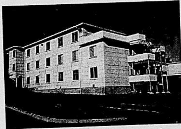
Photo 4.2.61 Building 224 east facade egress stairs
