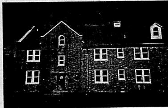
Photo 4.2.58 Building 26N entrance
