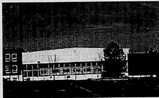
Photo 2.4 Building 30 in Activity Area 3
