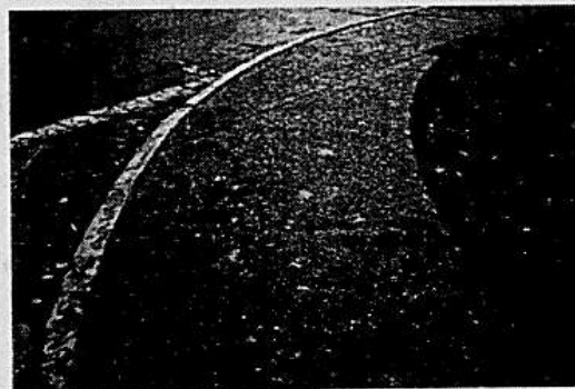
Photo 4.1.4.2 Exposed aggregate sidewalk at Sand Point
