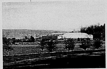
Existing Navy fields and former Navy Commissary. The Commissary is scheduled for demolition.
