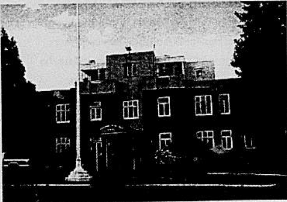
Photo 4.2.3 Former headquarters building
