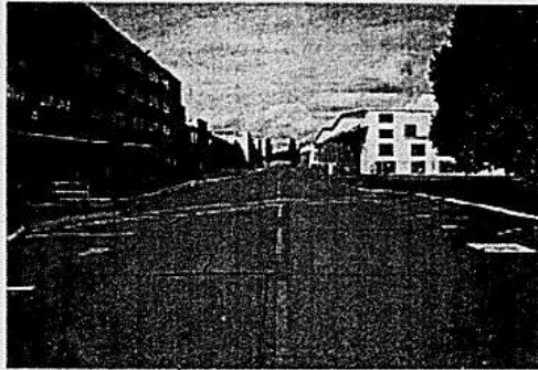
Photo 4.1.3.1 Looking north through the Sand Point and NOAA hangar buildings
