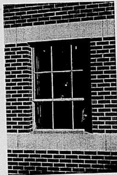
Photo 4.2.55 Building 47 metal framed windows
