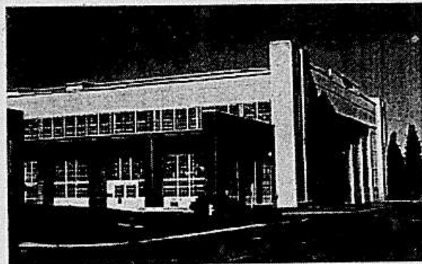
Photo 4.2.22 Building 2 side windows
