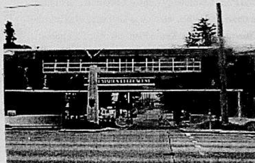
Photo 1.1 Main entrance at Sand Point.
