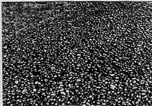
Photo 4.1.4.4 Typical existing exposed aggregate surfacing
