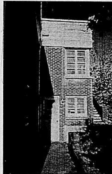
Photo 4.2.64 Wood & brick facade
