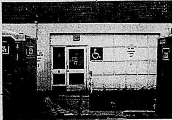
Photo 4.2.4 Existing barrier-free entrance
