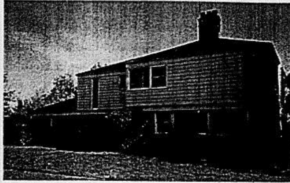
Photo 4.2.63 Typical street facade
