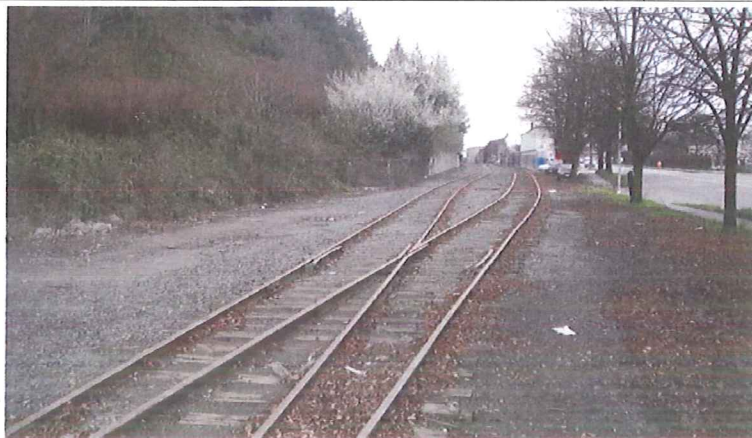
A portion of track north of South Snoqualmie Street is a railroad switch turnout.
