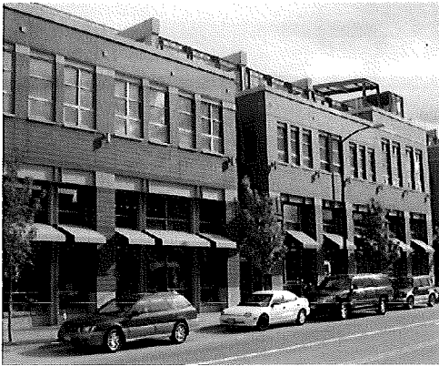
Active uses wrap a parking garage Land Use Code provisions require that aboveground parking be set back behind the facade, and that 80% of the above-ground parking be wrapped in habitable residential or non-residential space. (Photo: Kyle Grading)
