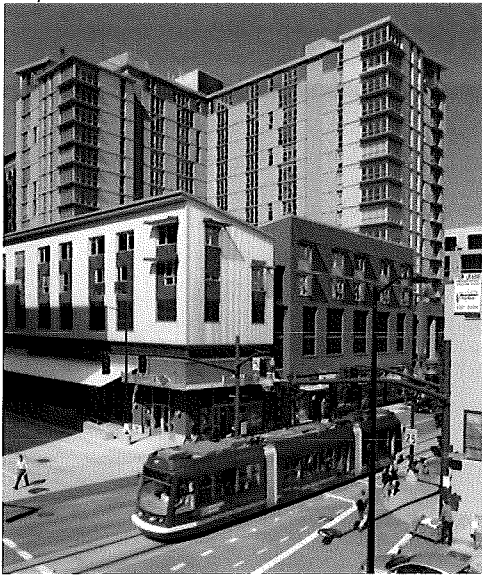
Differentiated massing and housing types This building incorporates highrise flats, courtyard-level townhouses, concealed parking, and street-level retail, all within a single block. Massing and facade design differentiate the housing types, reduce the bulk of building, offer a consistently activated street-edge, and create a balanced formal composition of the block. (Photo: Gregg Galbraith; Design: GGLO)
