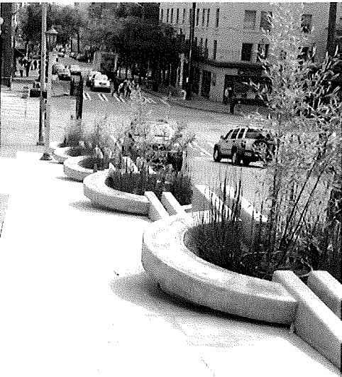
Cascading stormwater feature These cascading concrete pools and landscaping along Maynard in the International District are a good example of capturing and controlling the flow of stormwater on a sloping site in an artistic and engaging design. (Photo: City of Seattle)
