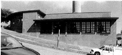
Yesler Terrace's historic steam plant The Yesler Terrace steam plant supplied heat to the original housing development, but was shut down due to failing distribution pipes. Designated as a landmark, SHA plans to renovate the facility for educational programming. (Photo: SHA)
