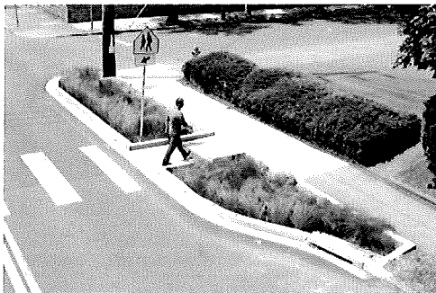
Curb bulb rain gardens Widened planting strips in the right-of-way provide an opportunity for stormwater management as a distinctive streetscape feature. (Photo: Portland Bureau of Environmental Services)
