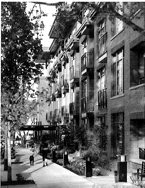
Finely scaled building features and rhythm This building increases the level of detail below 30 feet in height, using operable windows with divided panes, natural and durable materials, and pedestrian lighting. Window headers are expressed with brick soldier courses. (Design: Ankrom Moisan Architects)
