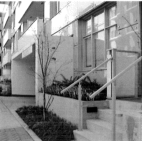
Appropriate edge for partially underground parking This terrace sits above a parking deck that extends above the sidewalk. The exposed portion of the parking is concealed by low walls and planting, which meets the requirements of SMC 23.75.180 for screening partially underground parking. (Photo: GGLO)
