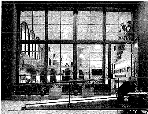
Access, visibility, and character Barrier-free access accommodates all users, railings and plants add texture to the building edge, low sills and a high level of transparency increase visibility, and high quality materials and rhythm create a pleasing facade. (Photo: Mathew Millman Photography; Design: Jones|Haydu)
