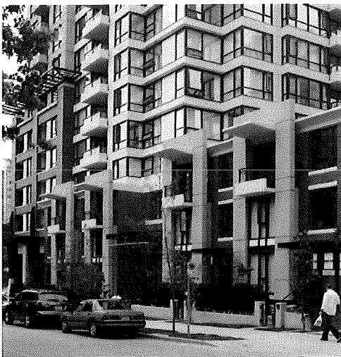
Neighborhood scale: appropriate articulation Articulated building facades respond to the neighborhood scale by adding visual interest to the street edge and breaking up the building mass. (Photo: GGLO)
