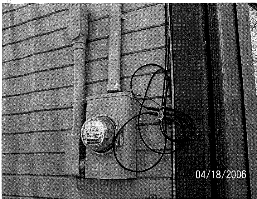
Figure 4: A Fully-Compliant Cable Drop Installation (Only 50% of drops inspected were compliant)
