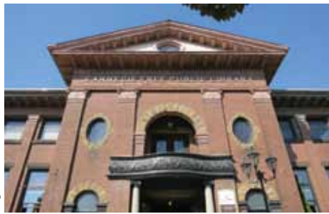
Ballard Carnegie Library, 2012
