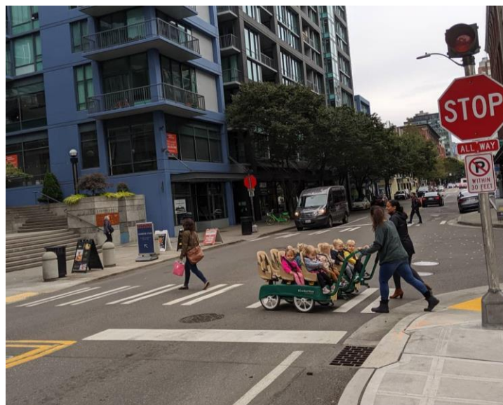
SDOT crews work hard to restripe crosswalks on a 4-year or better cycle to keep crossings bright and visible, helping our most vulnerable roadway users.
