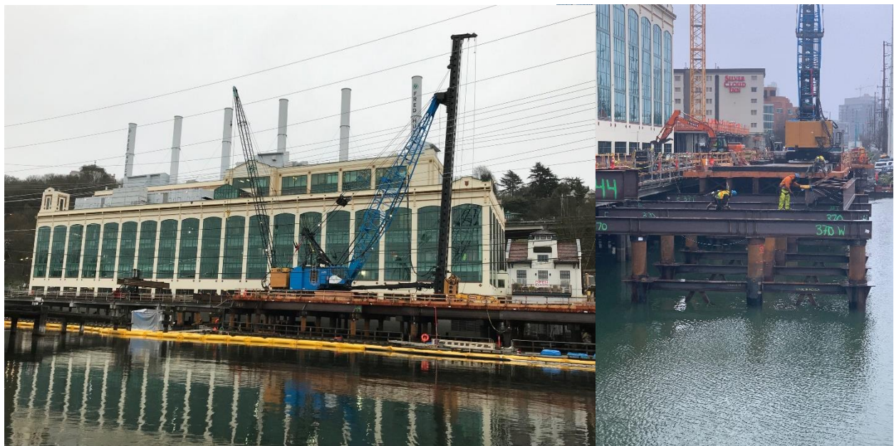
Construction is underway on the Fairview Bridge Replacement Project
