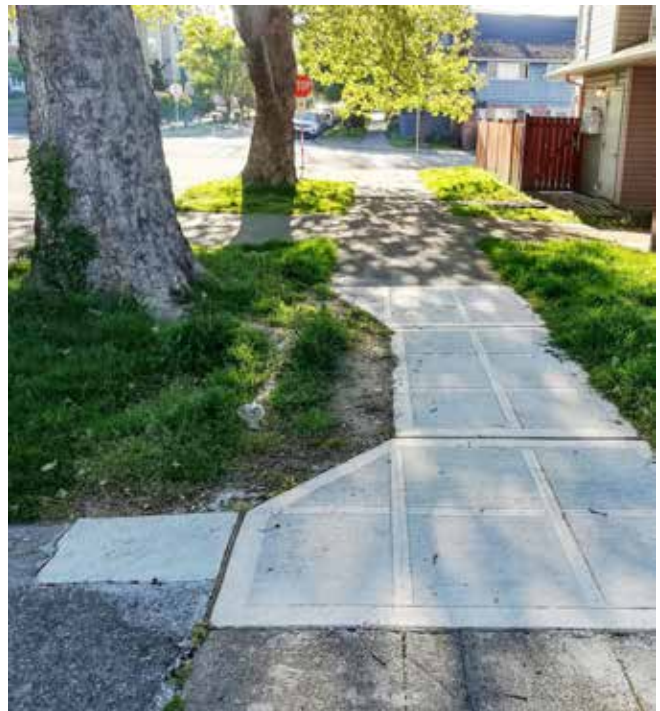
A new sidewalk rebuilt to meander around a mature street tree in order to reduce the likelihood of future uplift and impact to the existing root system
