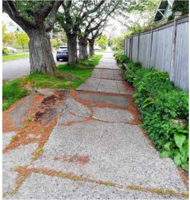
Mature tree roots uplifting a sidewalk, including shims that have succumbed to uplift.
