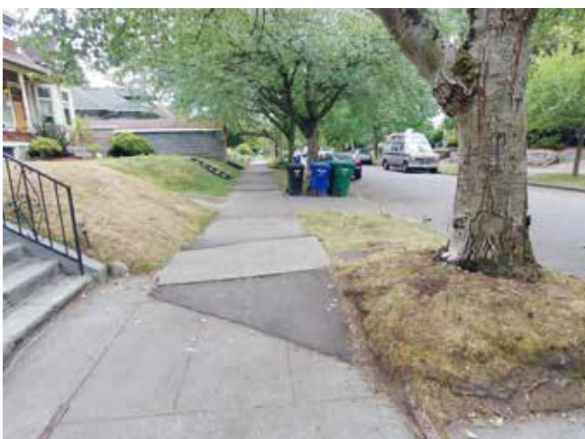
Shim addressing uplift from tree root
