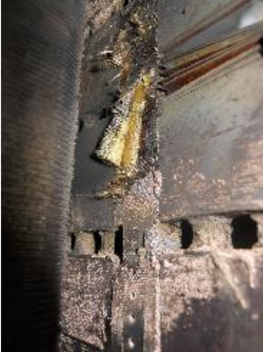
Unit 53: Separation of laminations
