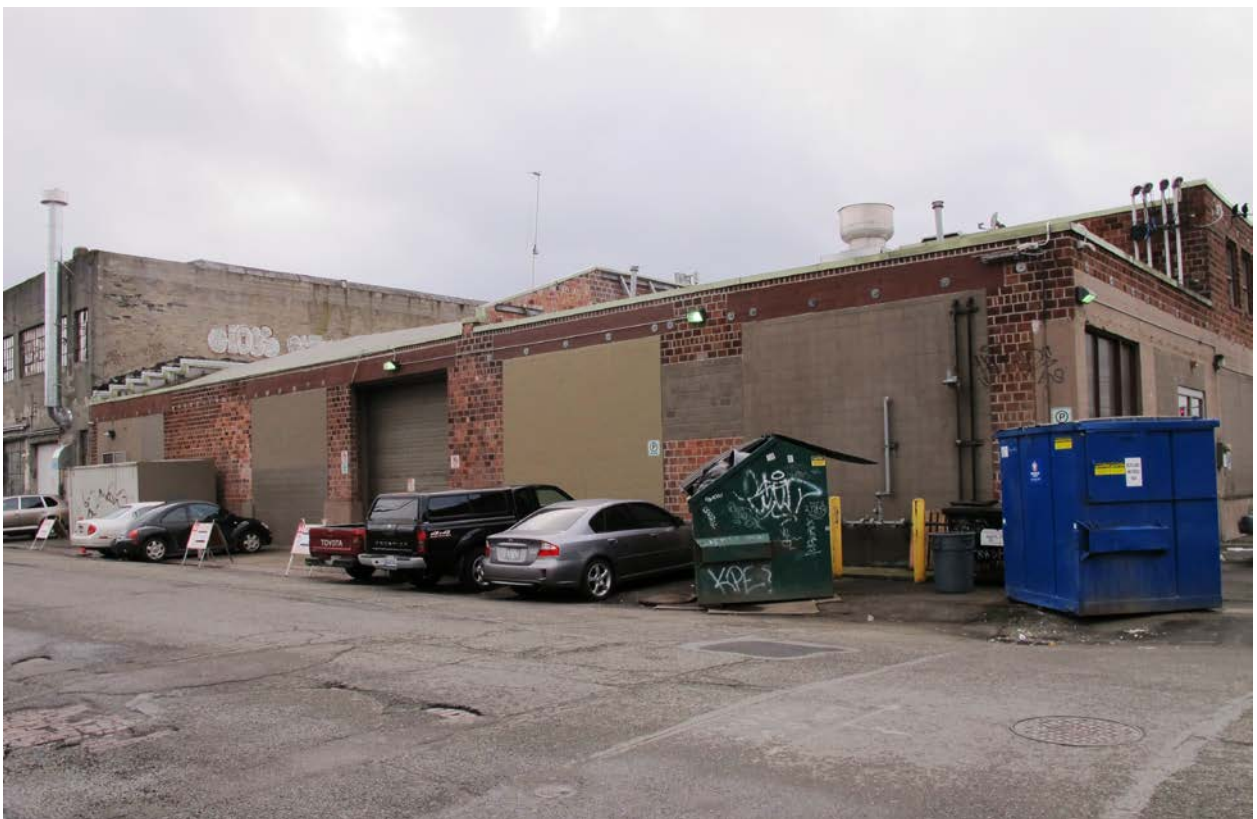
East elevation (facing Occidental Street)
