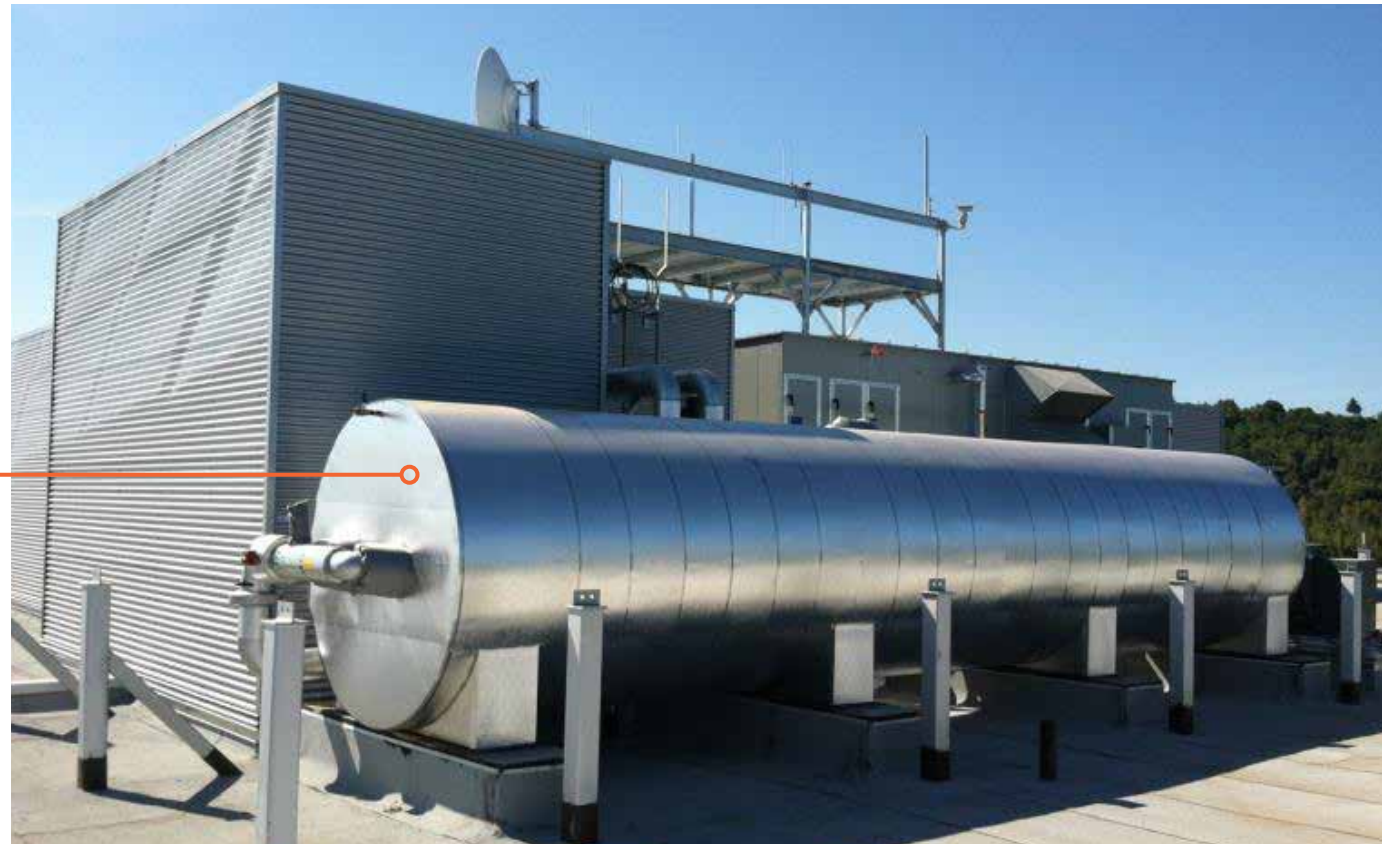
PHASE CHANGE THERMAL STORAGE AT FEDERAL CENTER SOUTH
