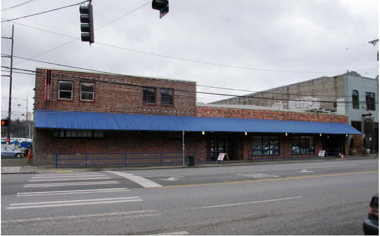
West elevation (facing First Avenue S.); note alterations to the right side of the facade (compare to 1937 photo).
