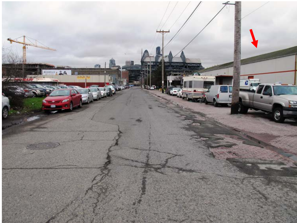
Neighborhood context: View north on Occidental Avenue S.; west elevation of subject building indicated by arrow.
