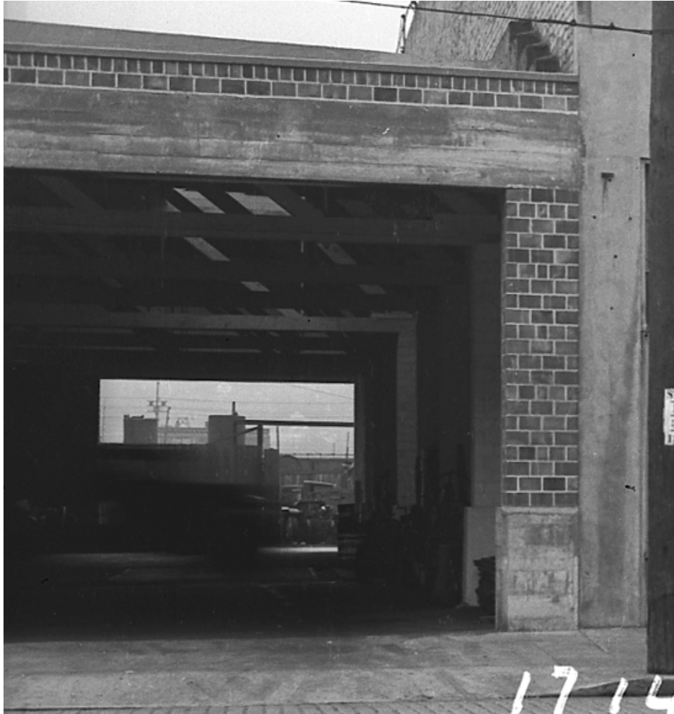
Detail of far south portion of west elevation, 1937 tax assessor photo of adjacent building, showing partial interior of the subject building, including roof trusses.
