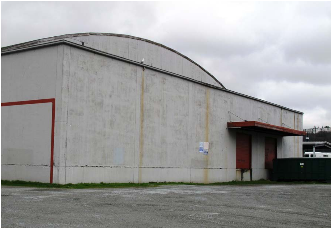
South elevation (facing S. Holgate Street)
