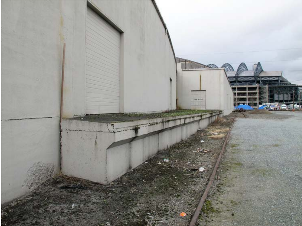
Detail, east elevation, showing former railroad-side loading docks
