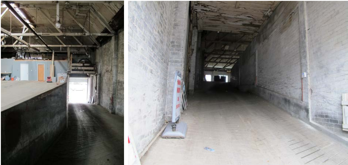
Ramp to second floor, accessed from east side of building.
