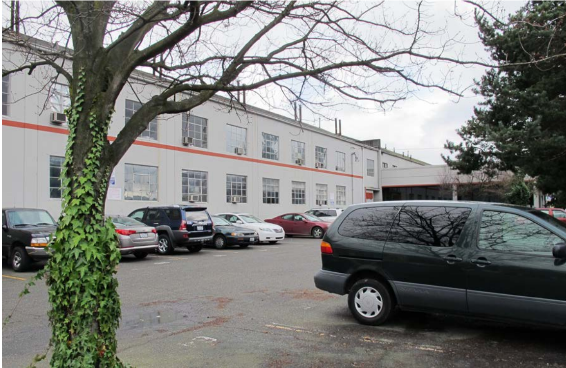
Looking southward, midblock on Occidental Avenue S., at the west elevation. Office addition at right.
