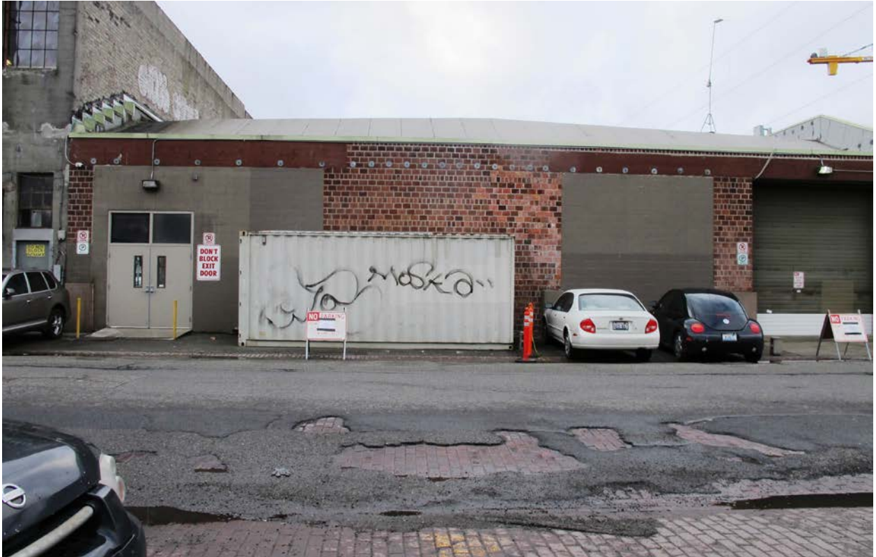
East elevation, south portion (facing Occidental Street)
