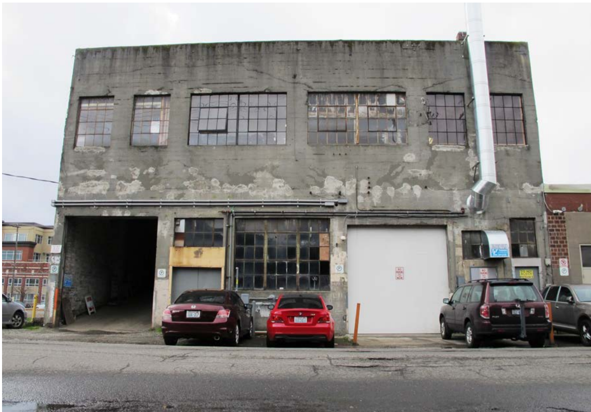
East elevation (facing Occidental Street). Open entrance at left gives access to an auto/truck ramp to the second floor.
