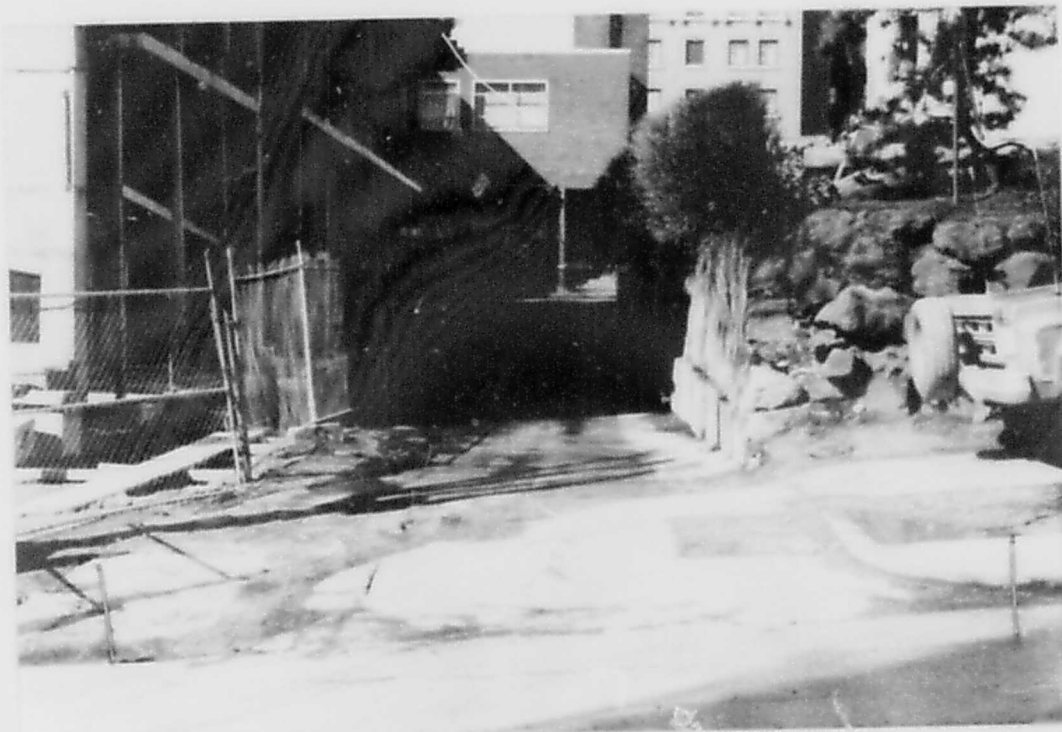
ALLEY FROM MARION STREET
