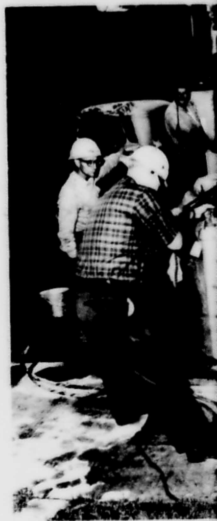
City Light crew plants distribution transformer in newly-made vault in Laurelhurst residential district, where underground utilities are replacing overhead service for over 1,000 homesites.
