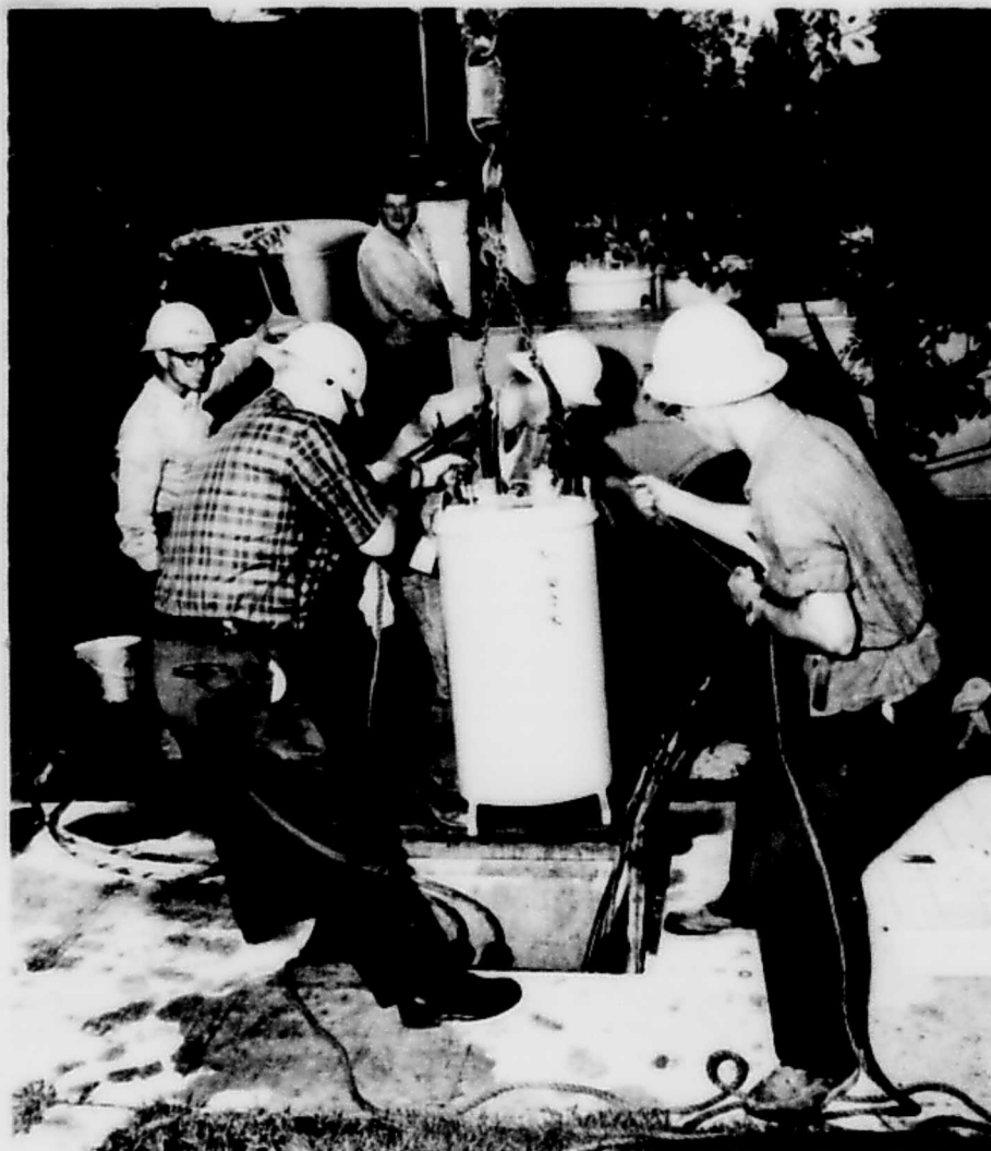
City Light crew plants distribution transformer in newly-made vault in Laurelhurst residential district, where underground utilities are replacing overhead service for over 1,000 homesites.
