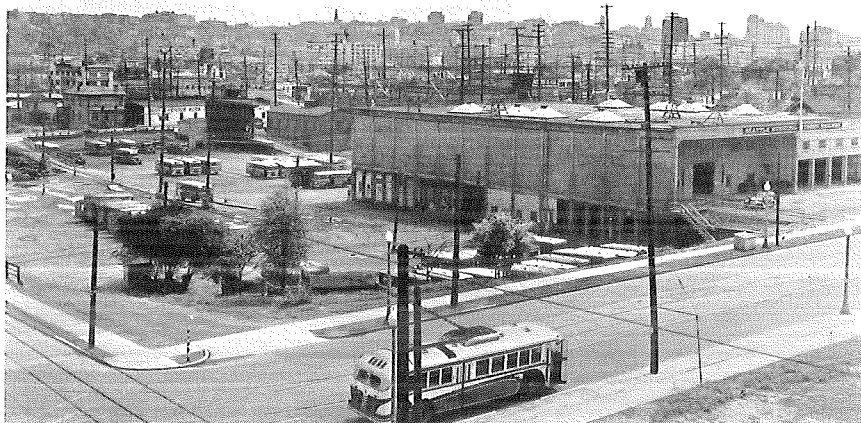
NORTH SEATTLE TERMINAL
