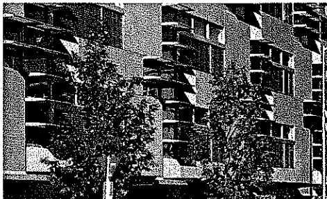
Louvers on the windows help moderate the amount of sunlight received into this building as do the deciduous trees.
