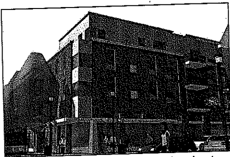
Example of a fourth floor upper level setback to reduce the apparent scale of new development
