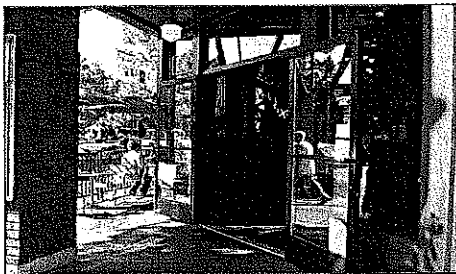
A well-marked, articulated building entrance that is oriented to the sidewalk and provides overhead cover.
