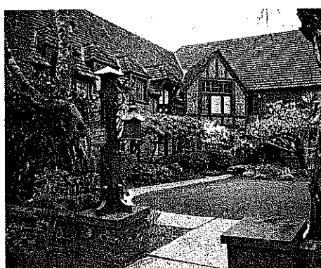
Maintain Landscape Traditions. Classic garden court-style apartment. Capitol Hill has an outstanding tradition of landscape design in its residential open spaces. Forecourts, intimate courtyards, terraces, and outdoor gardens contribute to an exceptional outdoor setting. New development should continue to build upon these traditions and qualities found within the local landscape.
