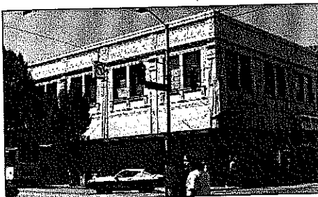
Examples of the classical detailing common on University Way.
