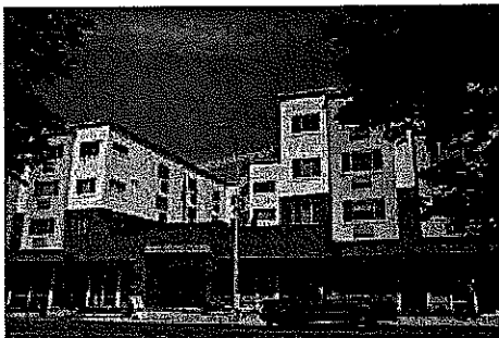
Where appropriate, consider using significant building setbacks and modulation to increase solar exposure to the site, and to preserve solar exposure to the surrounding area.
