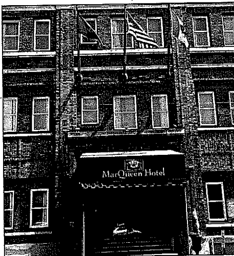
Decorative brick facades are important historic features in Uptown.
