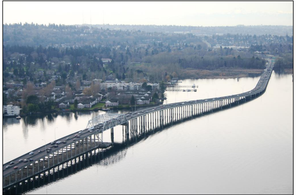
View of the existing west approach bridge, looking southwest towards Madison Park.
