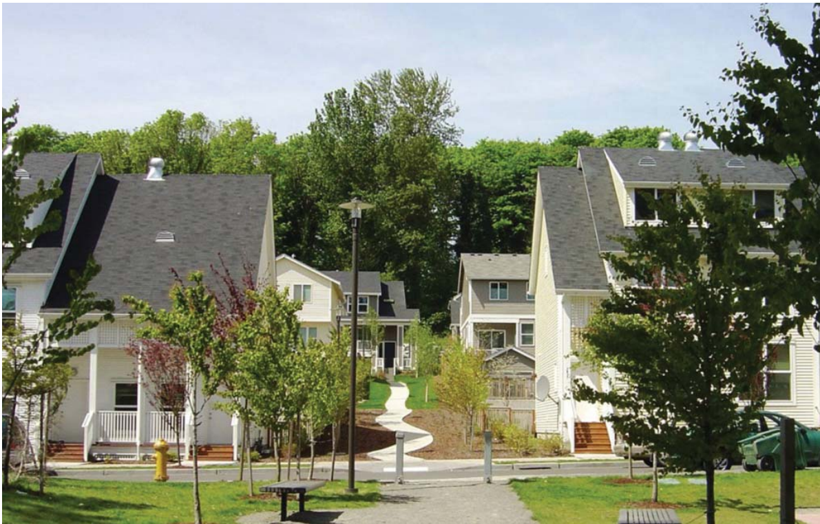
New Holly Transformation image credit: Seattle Housing Authority
