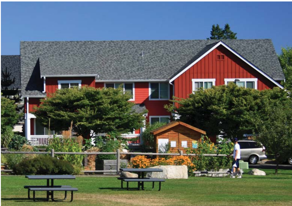
High Point Transformation; Seattle, Washington image credit: Seattle Housing Authority
